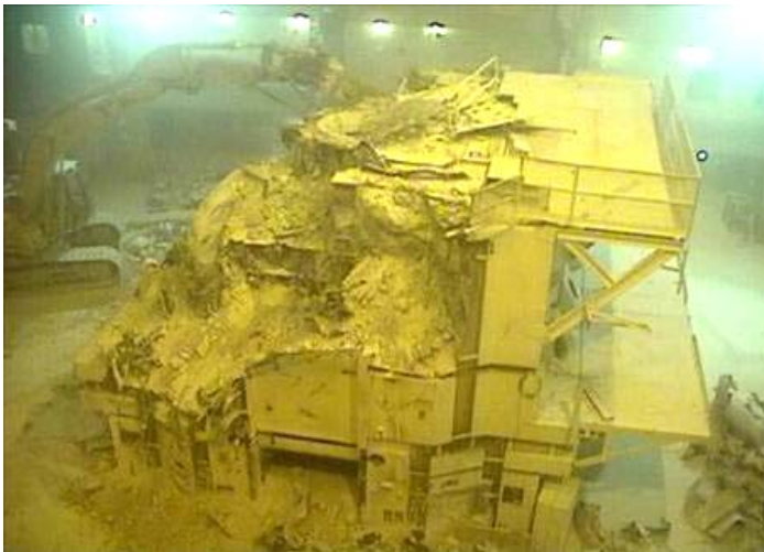
(Above) Demolition of the Materials Test Reactor at the Idaho National Laboratory
