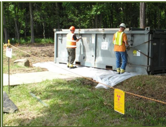
Packaging Contaminated Soil for Disposal
