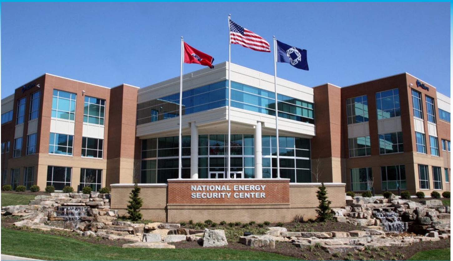
Clearing old, dilapidated facilities will expand the Science and Technology Park with new buildings such as the National Security Energy Center and the Commercialization Center.
