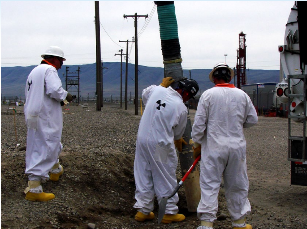
Workers begin excavation for a new Recovery-Act-funded interim moisture barrier at Hanford's TY Farm.
