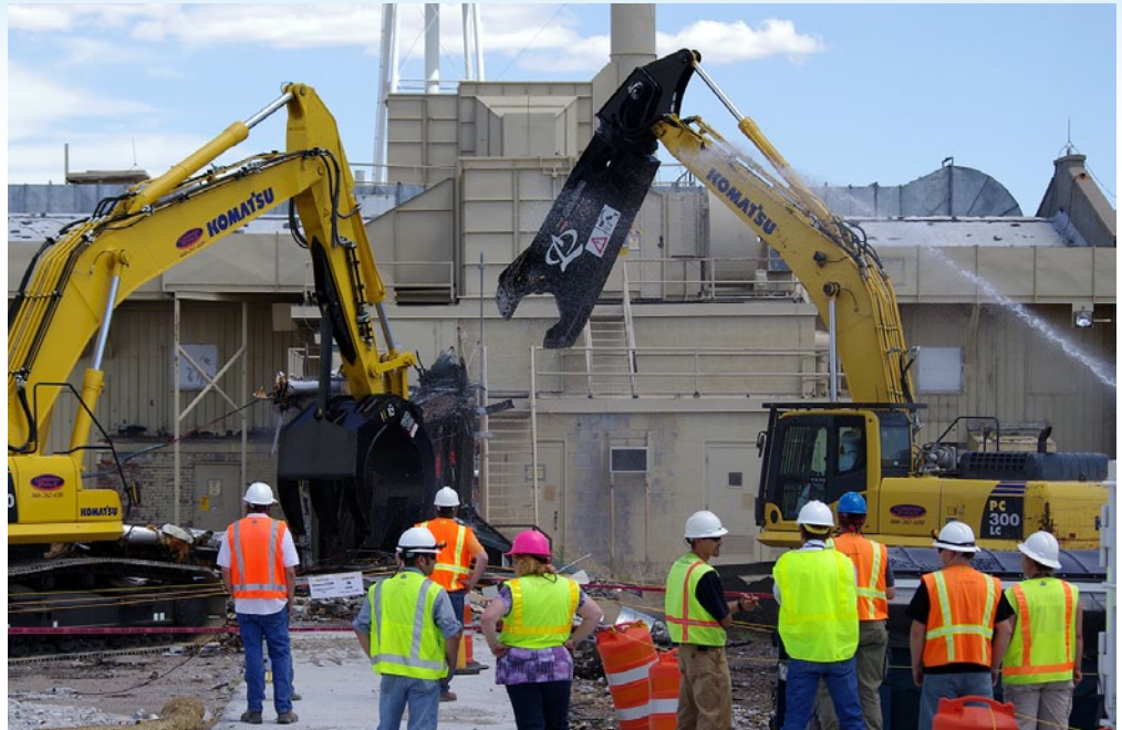
LANL safety and operations crews observe the demolition of the world's first full-scale plutonium processing lab. Known as “DP West,” the facility operated from late 1945 to 1978.
