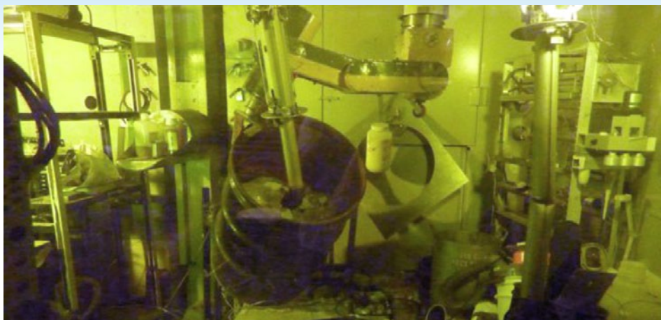
Debris is removed for packaging in Building 205, K-Wing, at Argonne National Laboratory.
