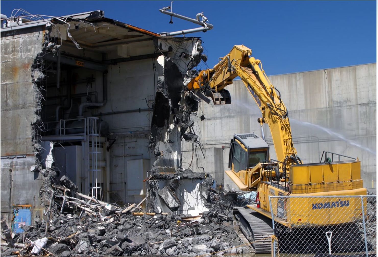
Workers demolish the 224-U facility, one of five ancillary facilities adjacent to Hanford's U Plant.
