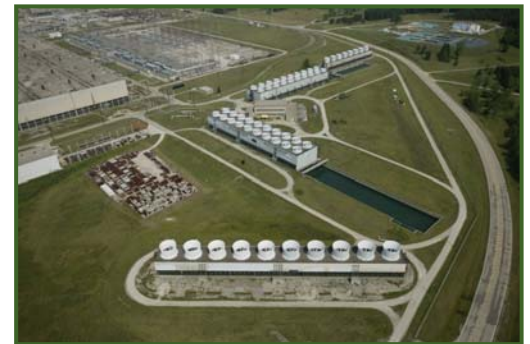
An aerial view of the X-633 Cooling Tower Complex at the Portsmouth Gaseous Diffusion Plant.
