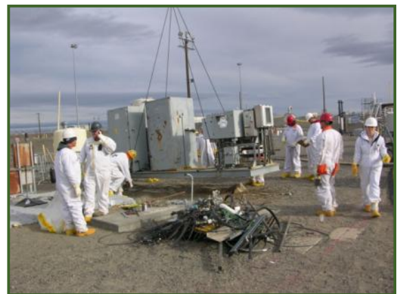
A PIC skid is removed from a Hanford tank farm.
