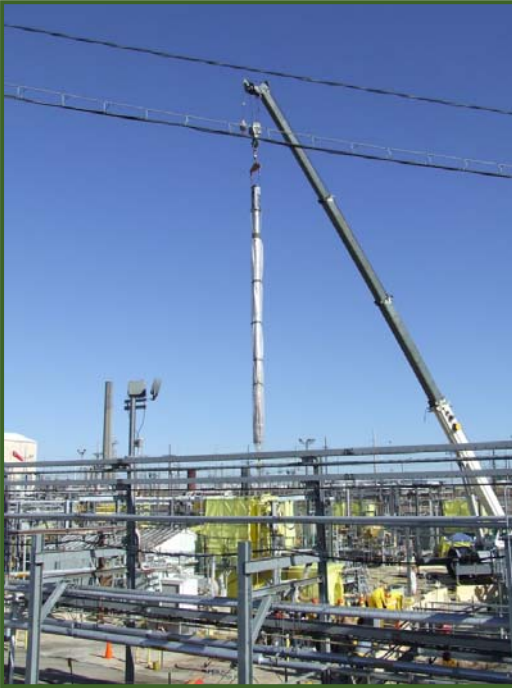
SRS workers remove a 50-foot submersible pump from waste Tank 5 during completion of tank operational closure.
