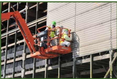
Workers remove asbestos exterior side panels from the cooling towers.
