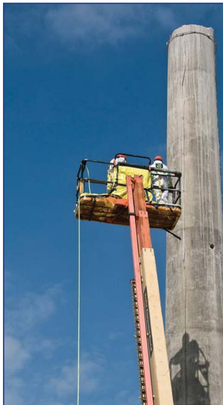
A man lift carries workers to the top of the stack, which will be reduced in size from 75 feet to 28 feet.
