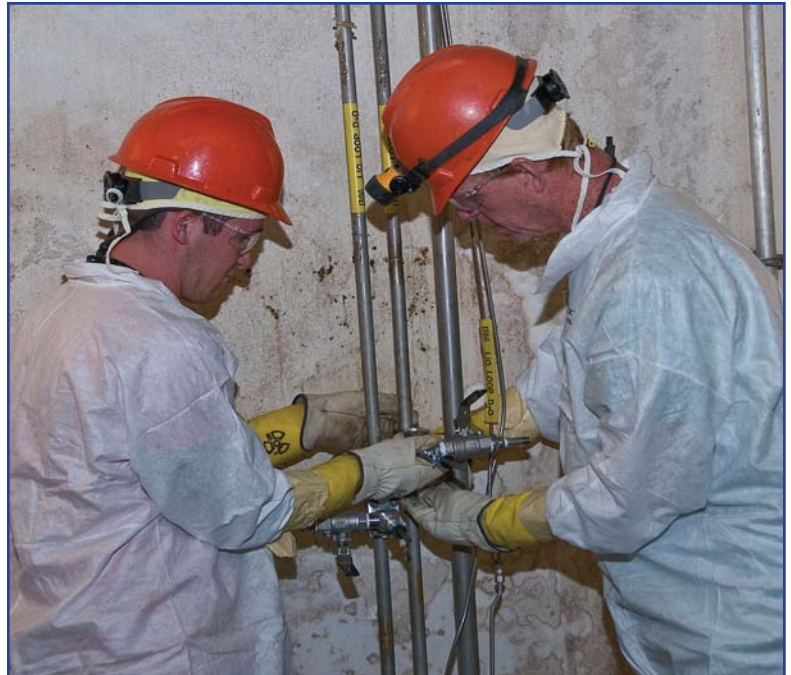
Workers install taps to drain fluids from old equipment before the next level of the reactor is enveloped by grout.
