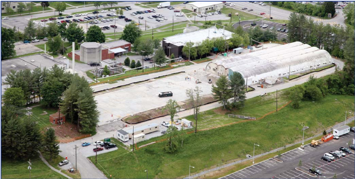
An aerial view shows the removal of the eastern side of the 2000 Complex. The western half will be down by November.
