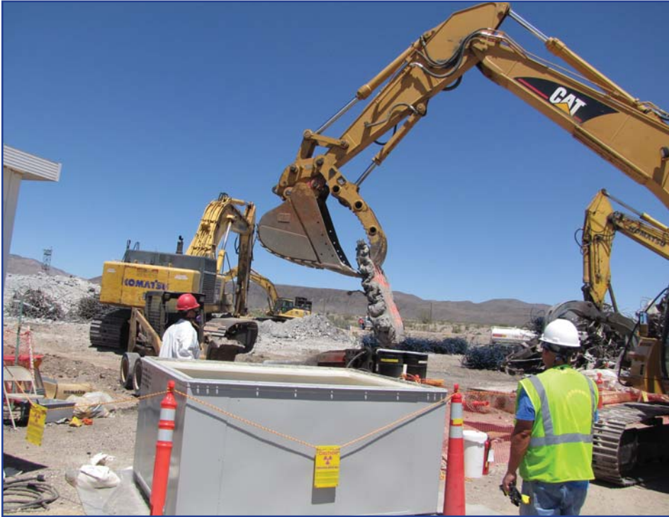
Workers remove mixed waste resulting from the demolition of the R-MAD facility at the Nevada Test Site.
