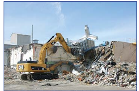
With a contaminated port removed, the processor pulls the rest of one of CPP-630’s rooftop ventilation plenums into the debris pile.
