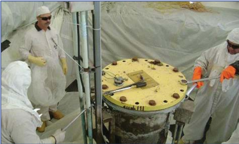
Construction workers remove bolts from the top of a cleanout box to prepare it for removal.
