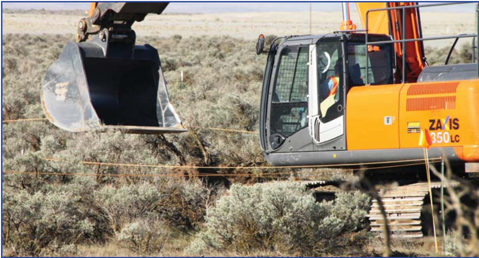
An excavator removes soil at the Hanford Site.
