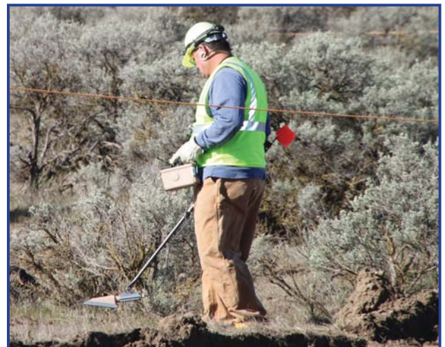
A radiological control technician surveys a section of the BC Control Area to confirm no contaminated soil was dispersed from an excavator that has just removed soil from the foreground. The spot requiring cleanup is one of several that CHPRC was able to pinpoint using radiological surveys last fall.
