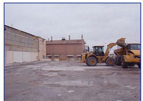
Debris cleanup occurs at the CPP-630 facility in May.
