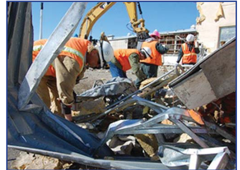
Radiological control technicians survey a pile of debris at CPP-630, a facility at the Idaho Nuclear Technology and Engineering Center.
