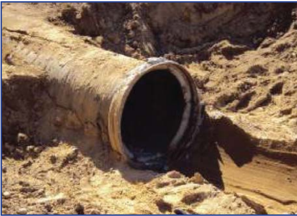
Excavation of underground air exhaust duct
