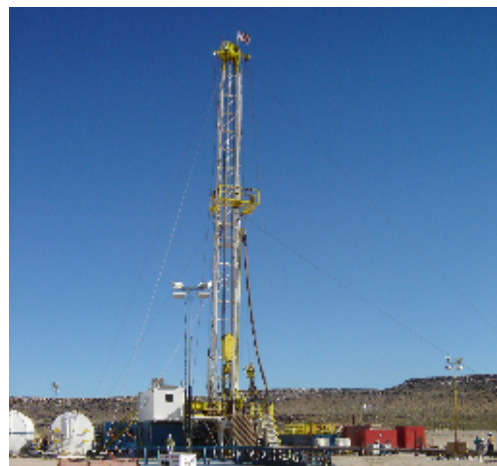
Drill rig mobilized at ER 20-8 at the Nevada Test Site.
