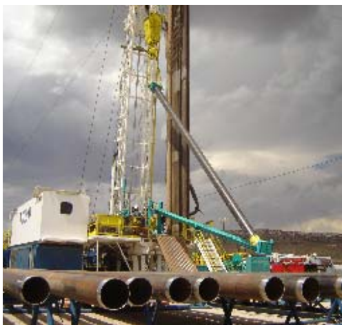
Casing is guided into position for installation in well ER 20-8 located on Pahute Mesa at the Nevada Test Site.
