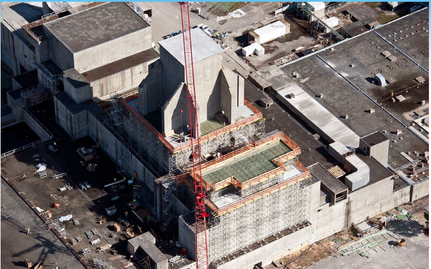
Workers prepare for roof modifications on portions of P Reactor at Savannah River Site that are expected to remain after facility decontamination and demolition efforts.
