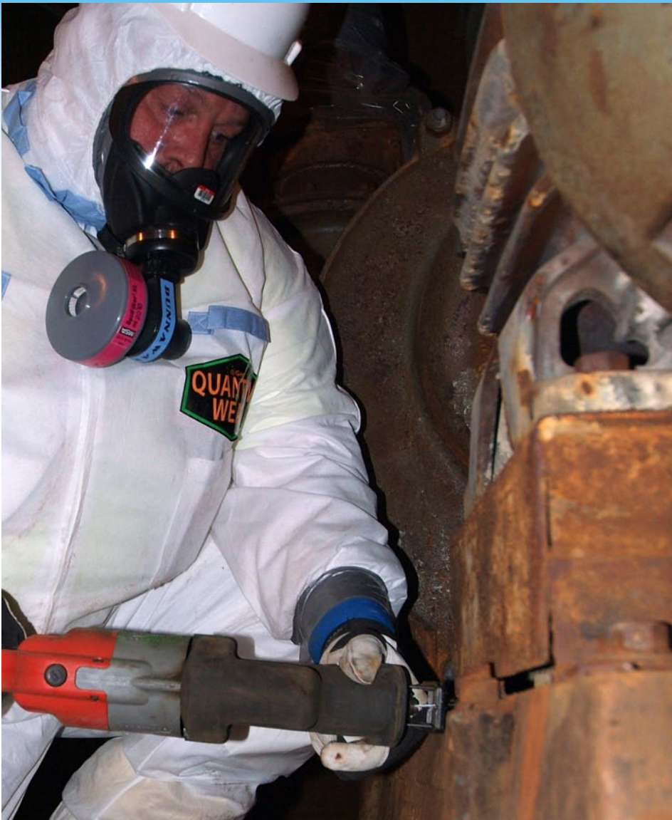
A Recovery Act worker saws a bolt loose so that a motor can be removed from the Feed Plant, which operated from 1957 to 1977. Uranium hexafluoride and fluorine were manufactured there.
