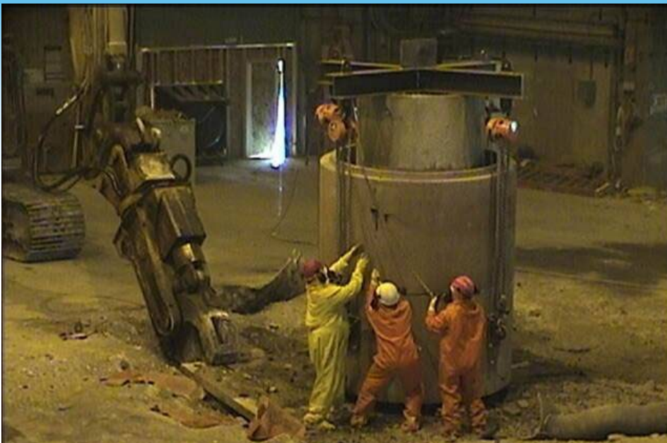
Workers install high-density concrete culverts to increase shielding around the Materials Test Reactor at the Reactor Technology Complex.
