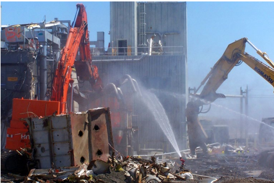
Workers demolish an ancillary facility near the U Plant processing canyon. They have removed five facilities – more than 53,000 square feet – to clear the way for a first-of-its-kind canyon demolition project, on target to begin in 2012.
