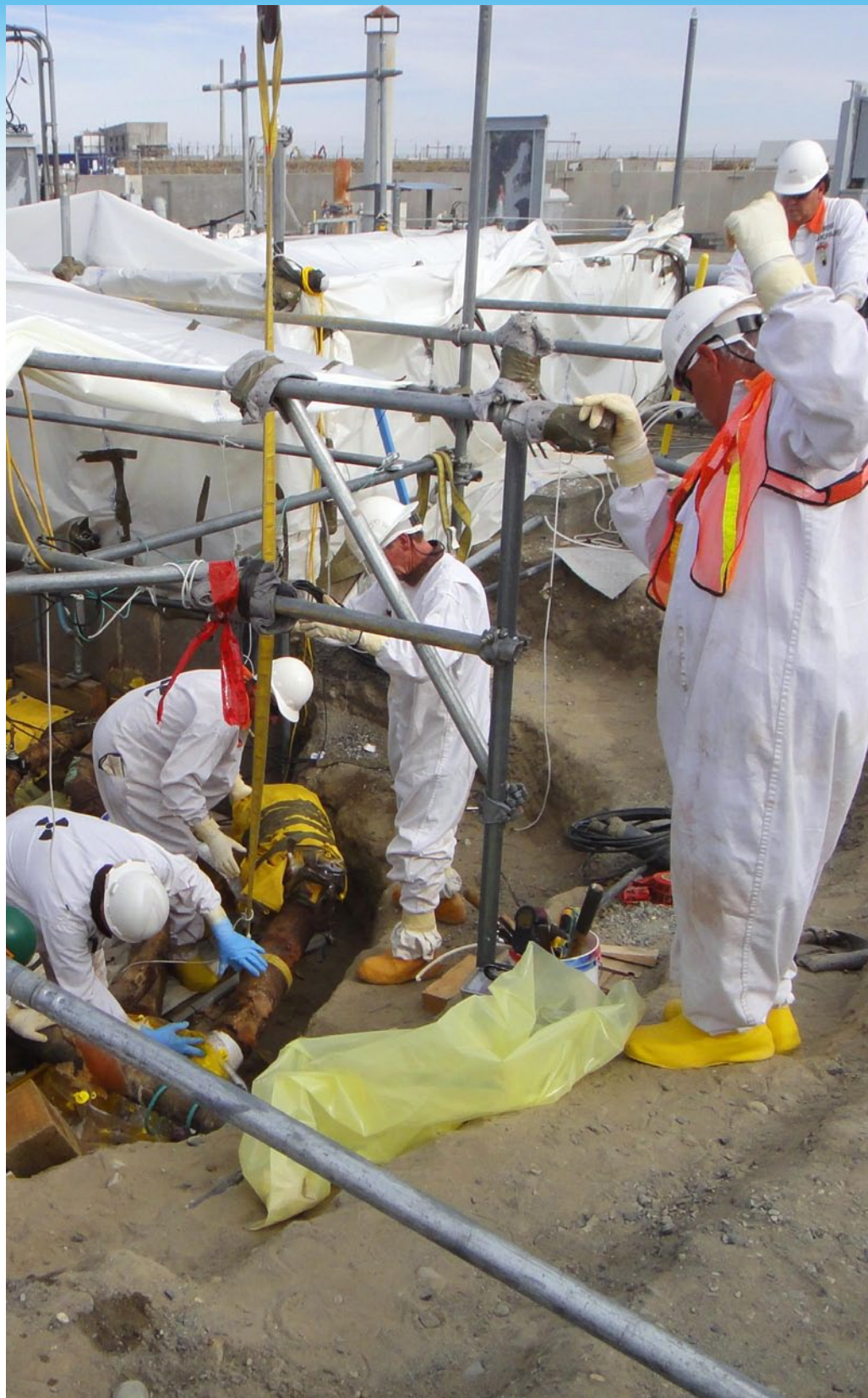
Workers remove the first portion of old pipe-in-pipe waste transfer lines from Hanford's SY Farm. The Recovery Act-funded project calls for a total of eight pipe-in-pipe waste transfer lines to be removed from the farm by the end of September 2011.
