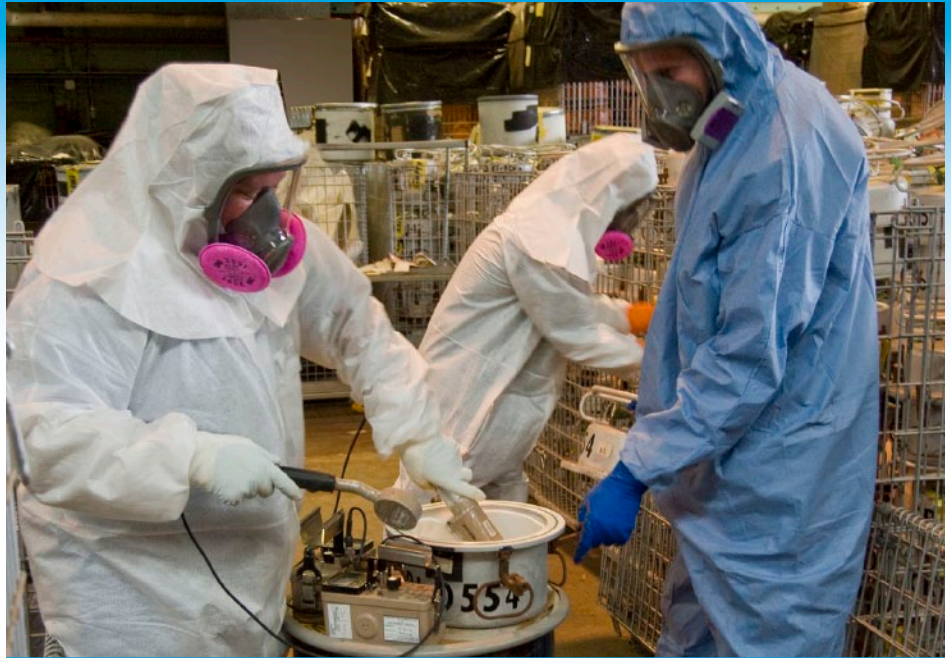
Recovery Act workers at Alpha 5 at the Y-12 National Security Complex at Oak Ridge, Tenn., survey waste as part of the characterization process to determine its proper disposition path.
