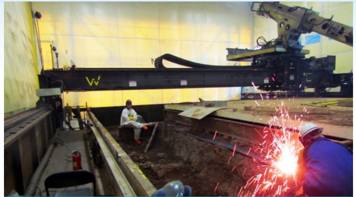
Recovery Act workers use a torch cutter to remove a reinforcing bar on the Brookhaven Graphite Research Reactor's bioshield.
