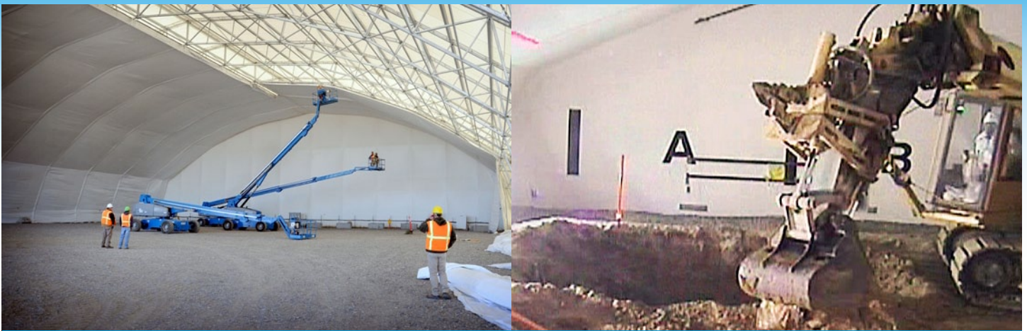
Workers install fabric inside the Accelerated Retrieval Project IV retrieval enclosure. Retrieval enclosures are designed to withstand sunlight, snow and wind and maintain a negative pressure inside.
