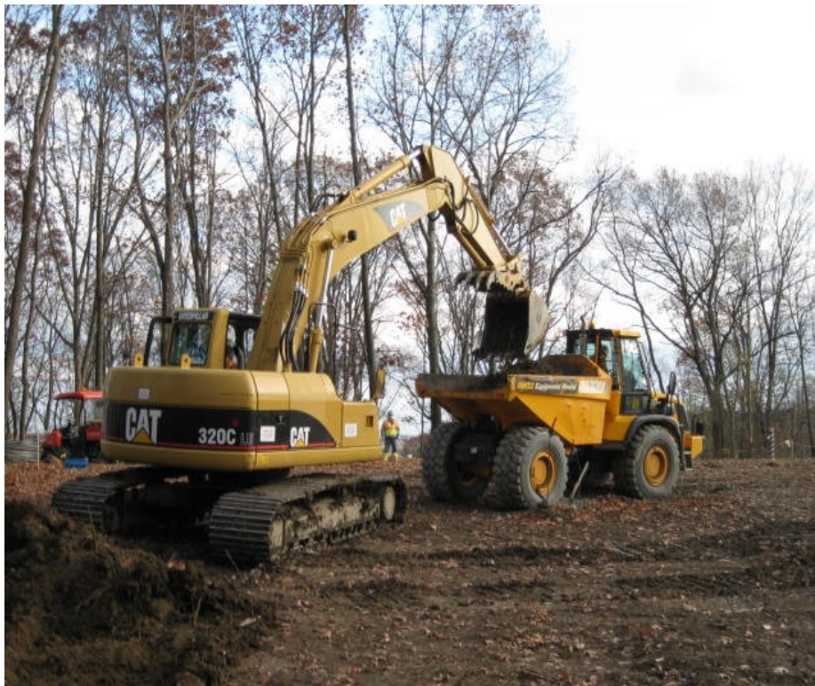
Soil removal operations underway at the North Field.
