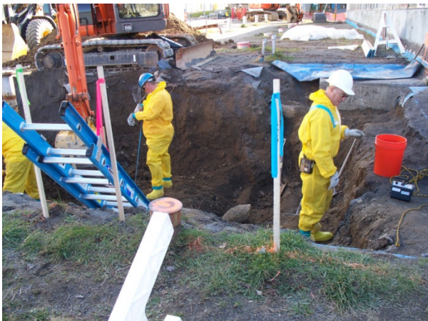
Excavation of soil over the H2 tank vaults.
