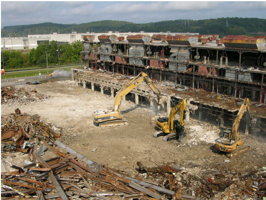
Much of the debris from the K-25 building demolition project is being shipped to the Environmental Management Waste Management Facility (EMWMF) at Oak Ridge.
