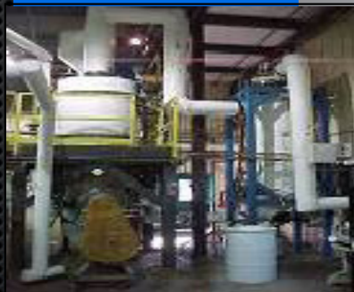
Fluidized Bed Steam Reformer
