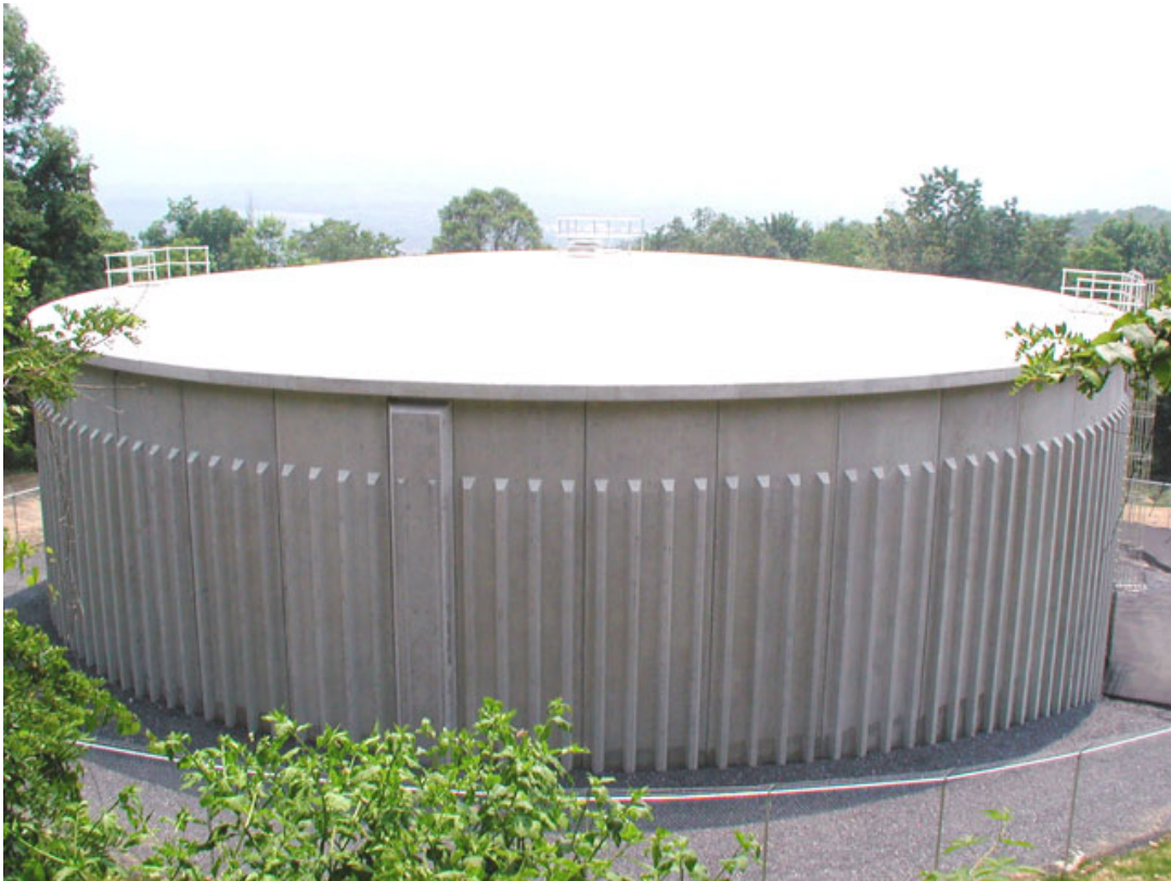
Figure 3.2-13: Vendor Example of Cylindrical, FDC Type Tank
