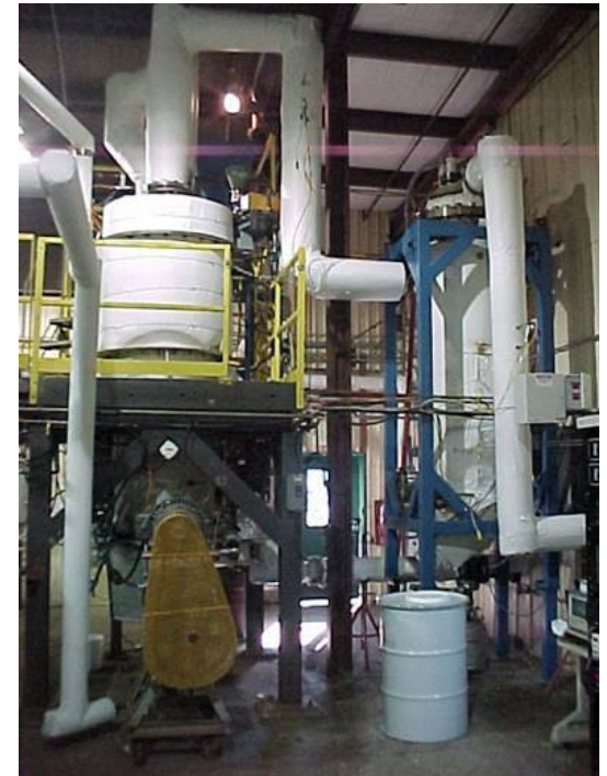
FBSR test facility at Hazen, CO
