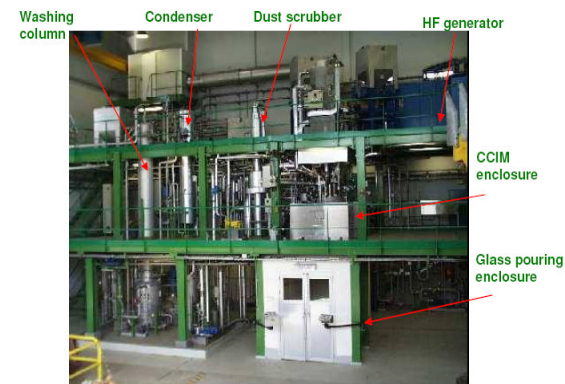
Figure 1: General view of the CCIM demonstration platform – CEA Marcoule
