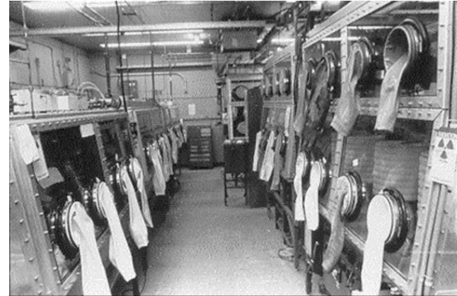
Glove boxes contaminated with GTCC Other Waste.
