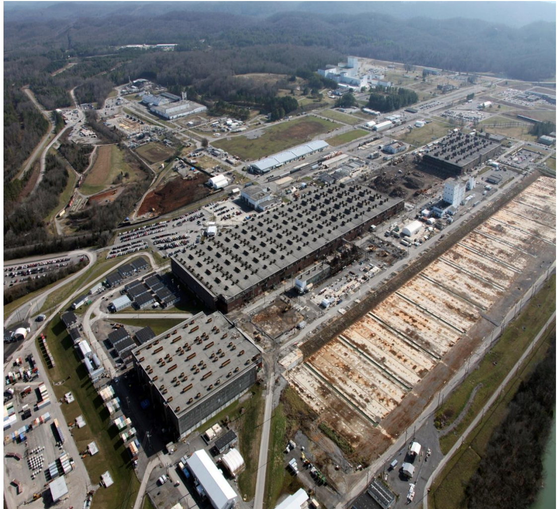
K-25 East Wing Demolition at Oak Ridge, TN
