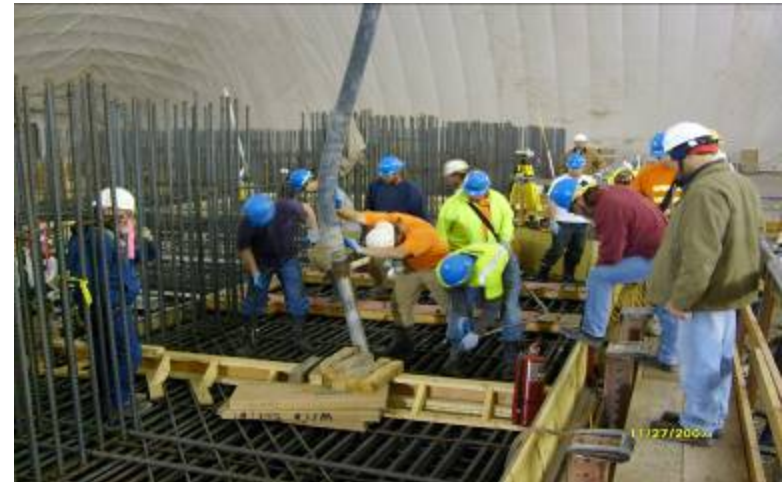
Concrete placement in basemat – November, 2007
