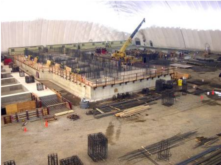
Process and Packaging Cell Basemat complete – January 7, 2008
