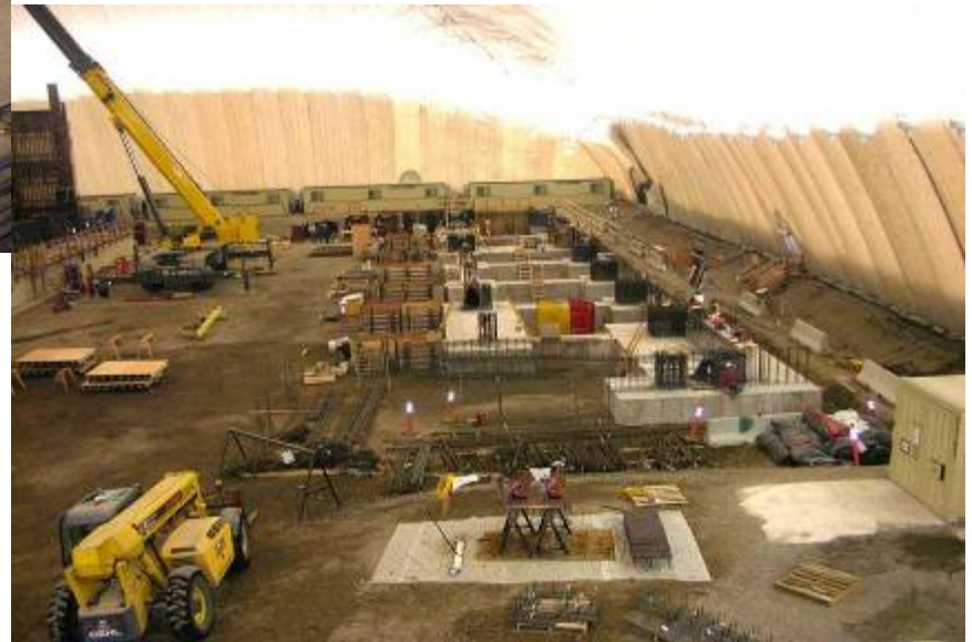
Mechanical Building Foundation Progress – February 25, 2008
