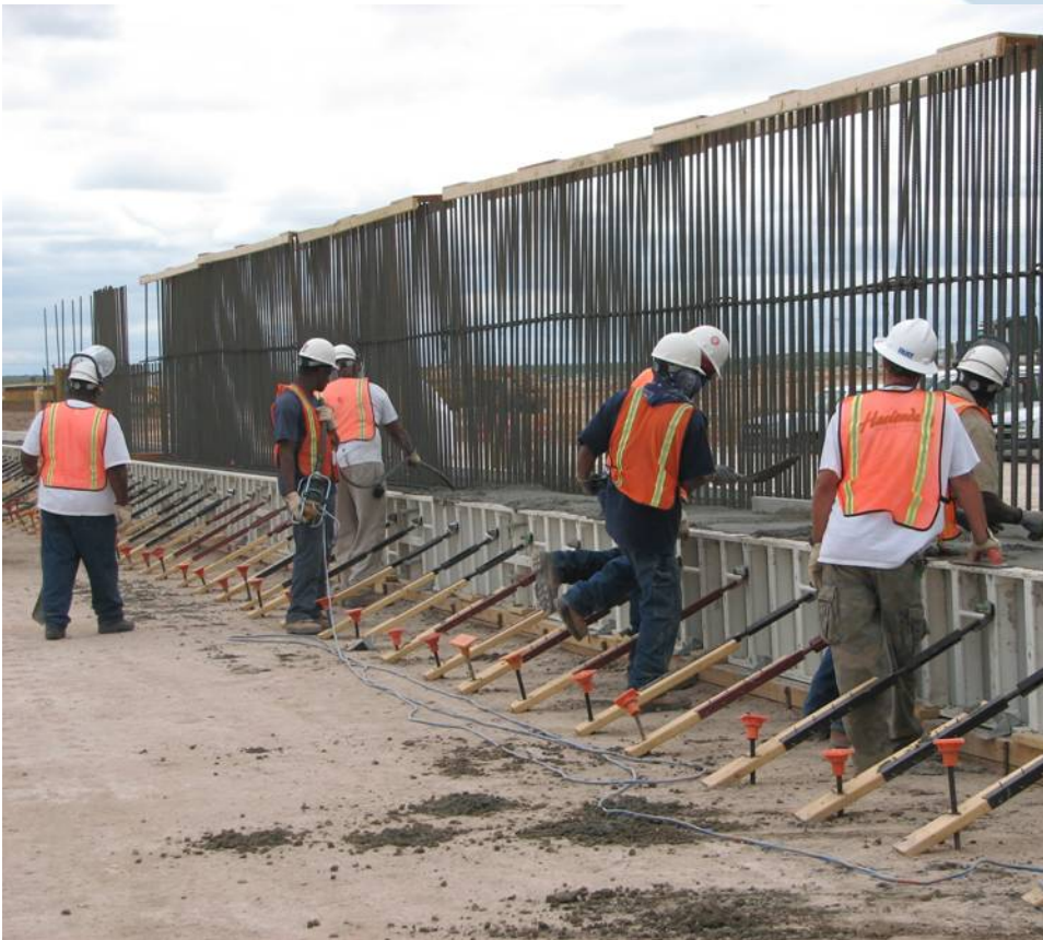
First NQA1 concrete placement at the National Enrichment Facility
