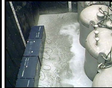
LLW Disposal Grouted in Vault
