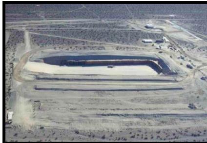
LLW Disposal Engineered Trench
