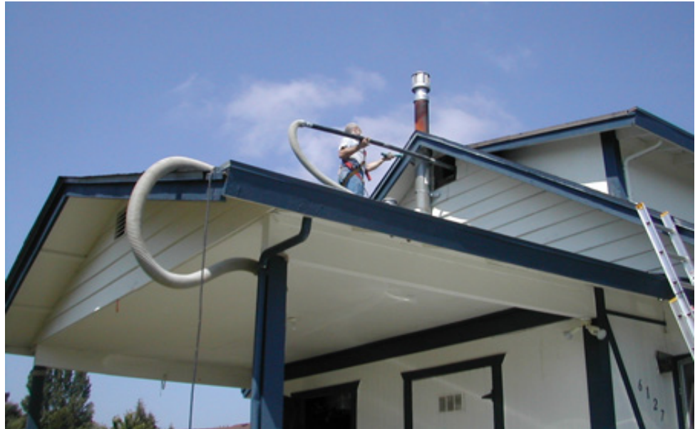
An energy auditor from Community Energy Challenge helps weatherize a home in Bellingham, Wash. | Photo courtesy of Sustainable Connections
