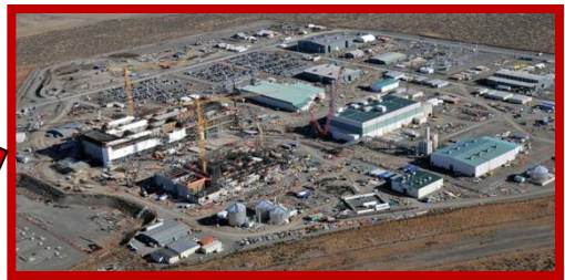
Hanford Waste Treatment Plant (WTP) ($690M)
