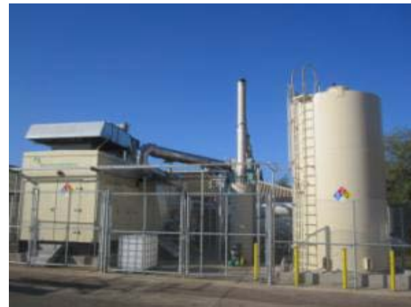
New CHP system at Manele Bay
