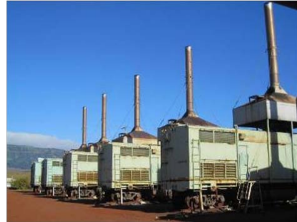
Older Diesel Engines on Lanai used for Peaking
