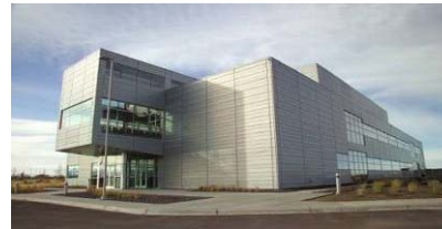
Center for Advanced Energy Studies (CAES)
