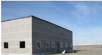
ATR Technical Support Building
