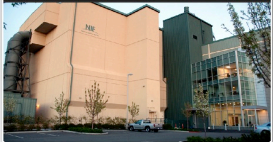
Outfitted Operational Support Facility
