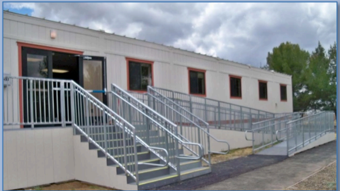
The interim HPC Innovation Center modular building
