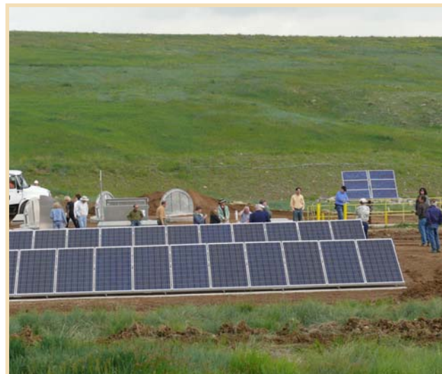
Stakeholders tour the Solar Ponds Plume Treatment System at the Rocky Flats, Colorado, Site.
