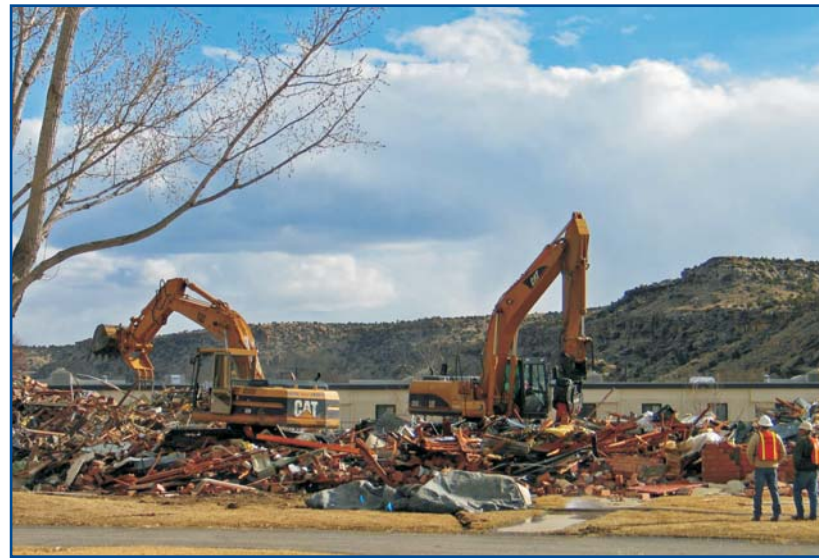
Demolition of laboratory at Grand Junction, Colorado, site
