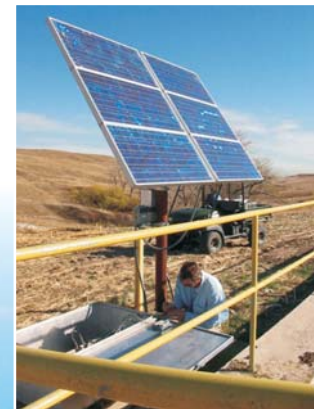
Rocky Flats, Colorado, Solar Pond Treatment System
