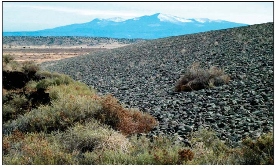
The Bluewater UMRCA Title II disposal site is in the Grants Mineral Belt of New Mexico. The main cell at Bluewater is the largest UMRCA cell managed by LM, covering over 400 acres (162 hectares). Mt. Taylor, a prominent peak in western New Mexico, is in the background.
