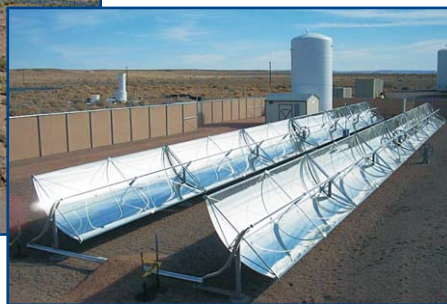
The parabolic mirrors focus solar energy to preheat the water to 170 degrees before it goes into the treatment system.
