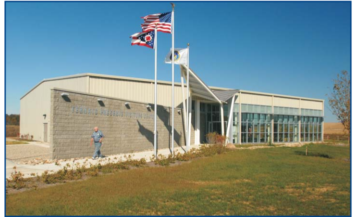
The high-efficiency windows in the Office of Legacy Management's Fernald Preserve Visitors Center provide natural light and passive solar heating. A green building also offers environmental, economic, health, and community benefits.
