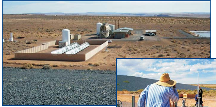
The solar hot water system is estimated to reduce the amount of electricity used to operate the Tuba City Site groundwater treatment system by 15 percent.
