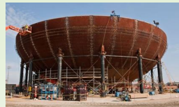
Vogtle Unit 3 Turbine Building Basement and Containment Vessel (Courtesy of Southern Company)
