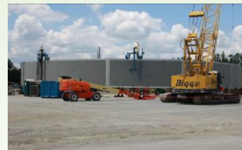
VC Summer Unit 2 Lower Bowl Assembly and Containment Vessel Ring (Courtesy of SCANA)
