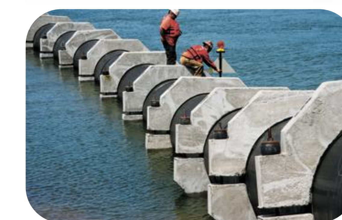
Pipe Laying Feasibility
