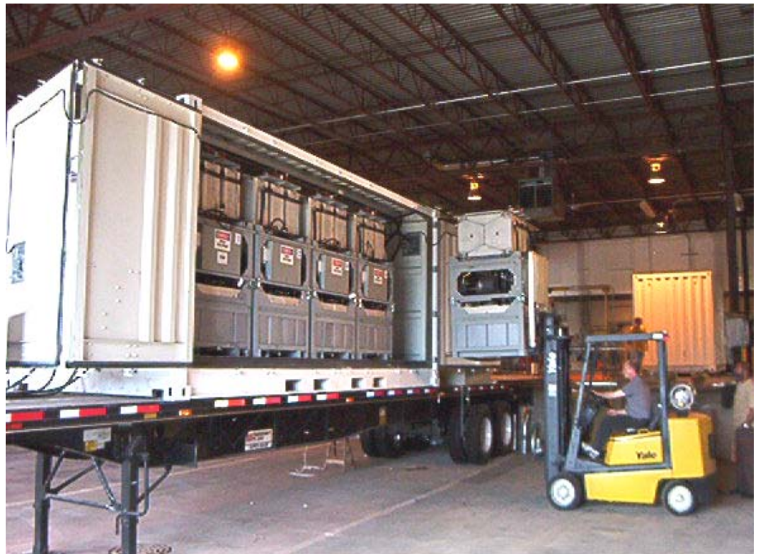
ZBB's 500 kWh system (10 - 50 kWh modules)
