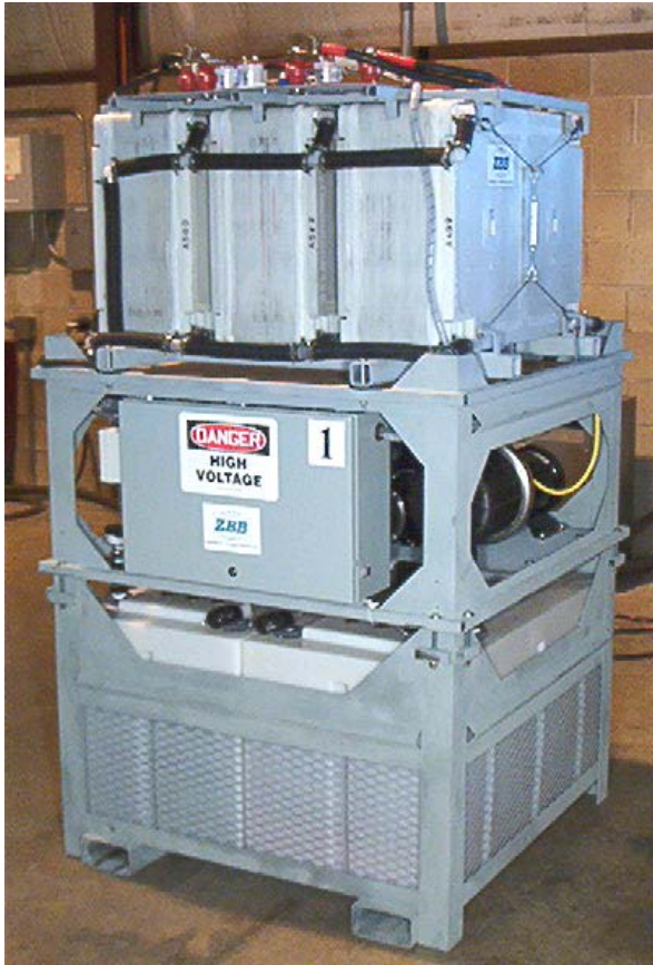
ZBB's 50 kWh module (3 stacks in parallel)
