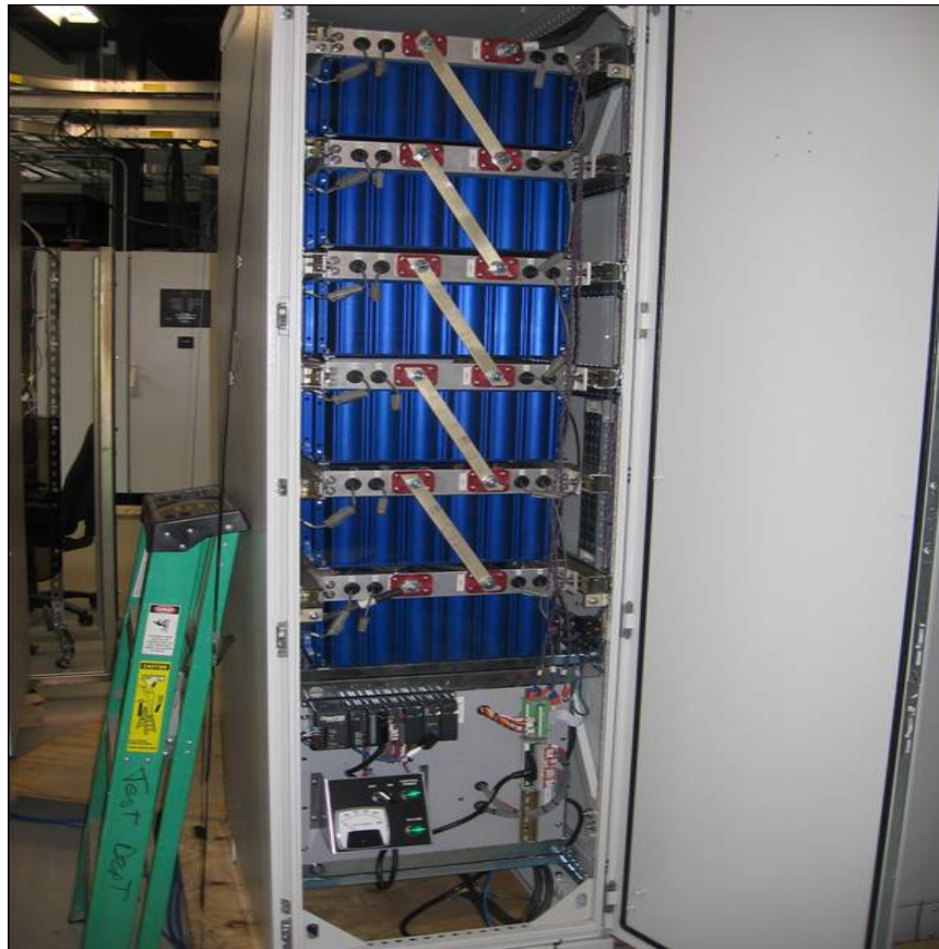
One of four ultracapacitor cabinets
