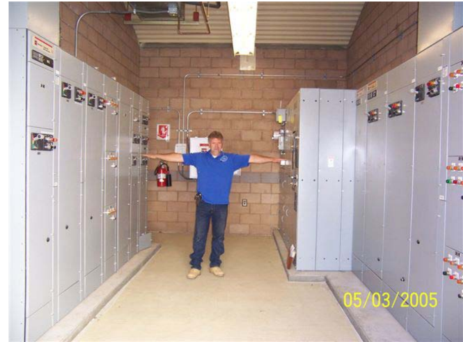
Existing Electrical Panels (no more room)
