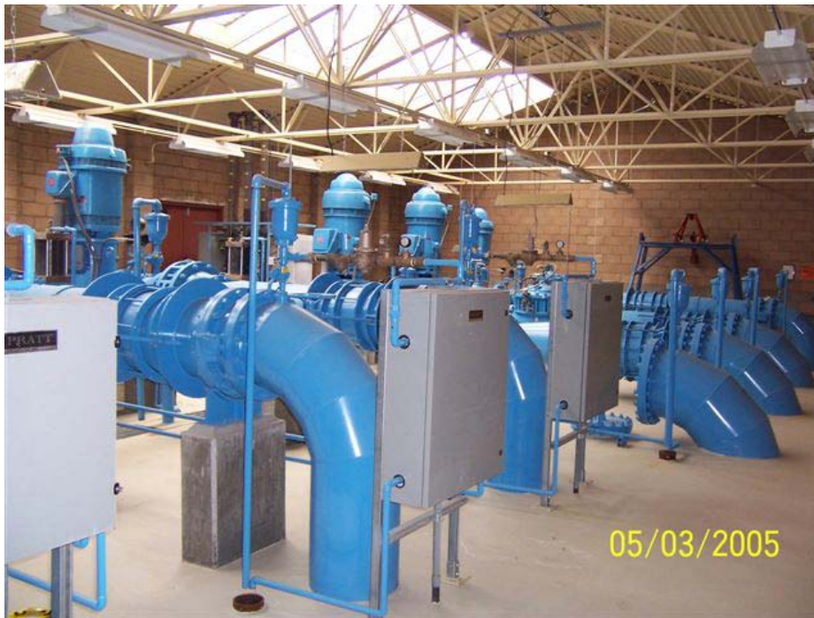
Loads: water pumps Good test but not typical
