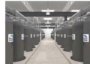
1st MW operational in commercial service
