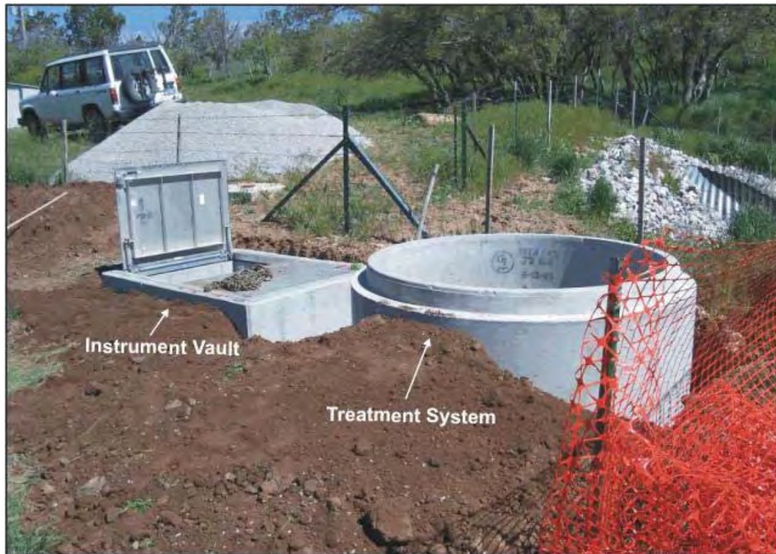
Figure 1. Photo of Instrument Vault and Treatment Cell TC1 Prior to Filling with Reactive Material. Water was pumped through the treatment cell from bottom to top.
