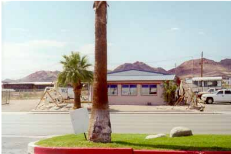
Photo 4: View of a building that may be removed due to realignment of U.S. 93 as part of Alternative B.
