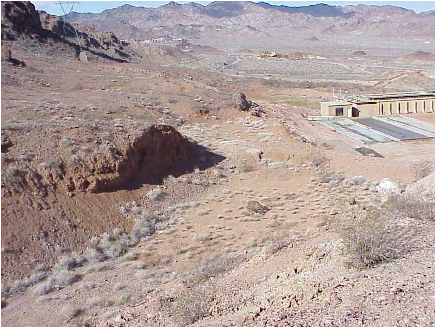
FIGURE 4-7 WASH CROSSING B-9 (CUTOFF AT WASTEWATER TREATMENT FACILITY) LOOKING NORTH - ALTERNATIVES B AND C BOULDER CITY/U.S. 93 CORRIDOR STUDY ENVIRONMENTAL IMPACT STATEMENT
