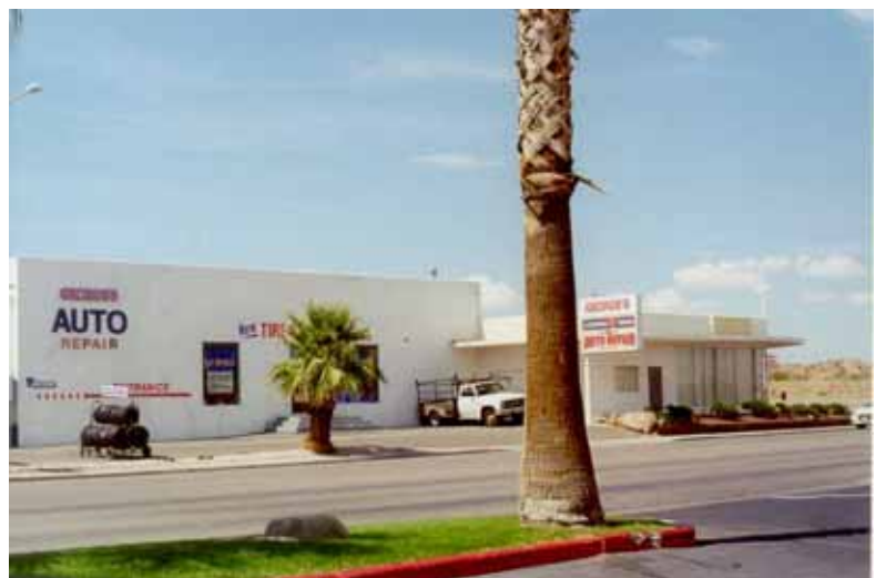
Photo 5: View of a building that may be removed (the smaller building to the right side of the tree) due to realignment of U.S. 93 as part of Alternative B.
