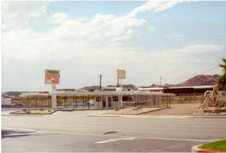
Photo 3: View of a building that may be removed due to realignment of U.S. 93 closer to the building as part of Alternative B.
