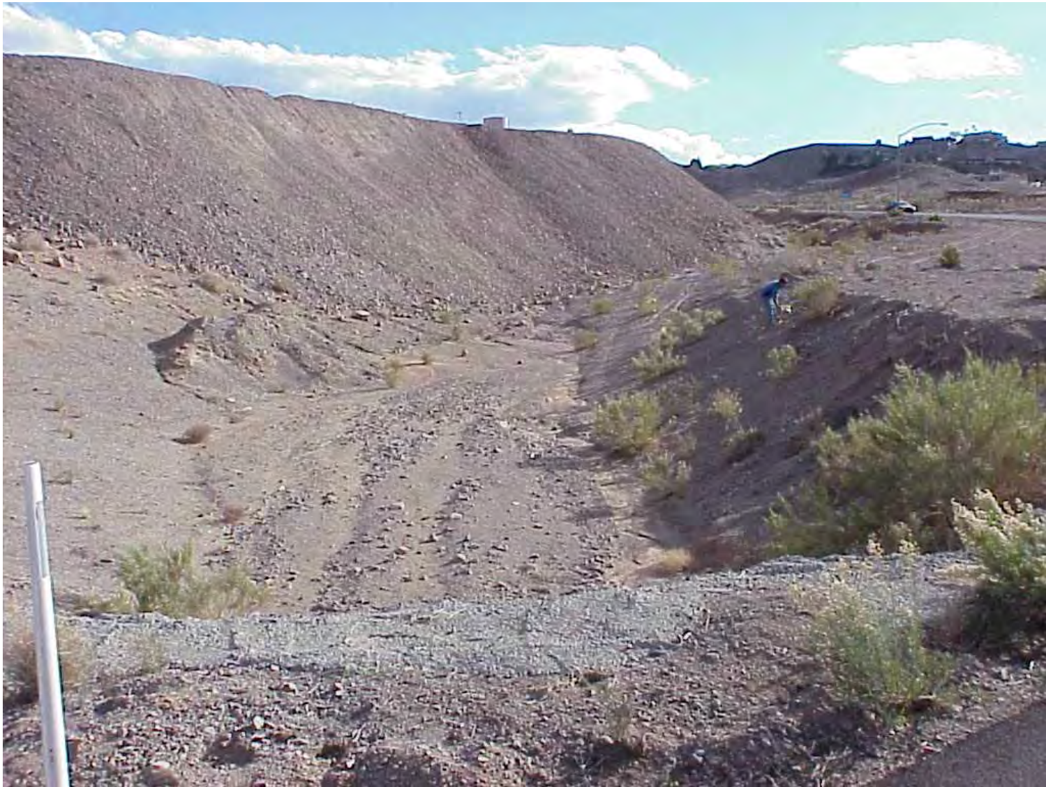
FIGURE 3-8 WASH CROSSING C-3 (U.S. 93 AT NEVADA WAY) LOOKING UPSTREAM BOULDER CITY/U.S. 93 CORRIDOR STUDY ENVIRONMENTAL IMPACT STATEMENT
