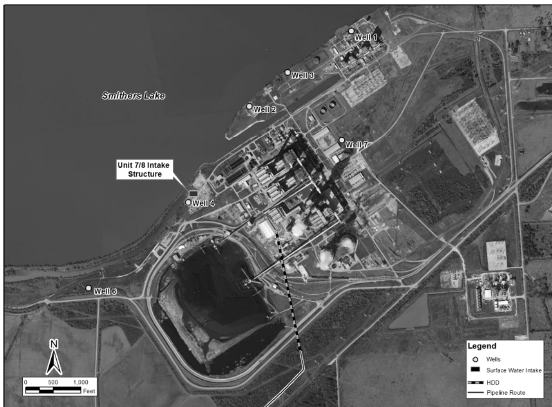
Figure 2-6. Existing W.A Parish Plant Water Supply Sources
