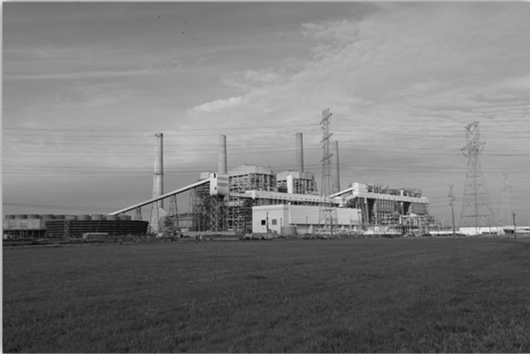
Figure 2-1. W.A. Parish Plant
