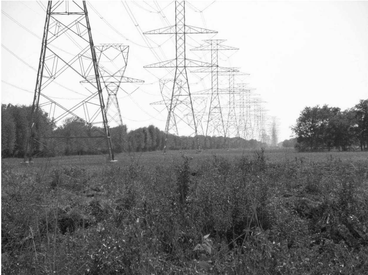
Figure 3.11-1. Typical View of the Proposed Pipeline ROW Along the CenterPoint ROW (Looking Southwest near FM 762)
