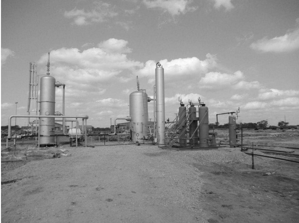
Figure 3.11-3. Existing Oil Field Equipment
