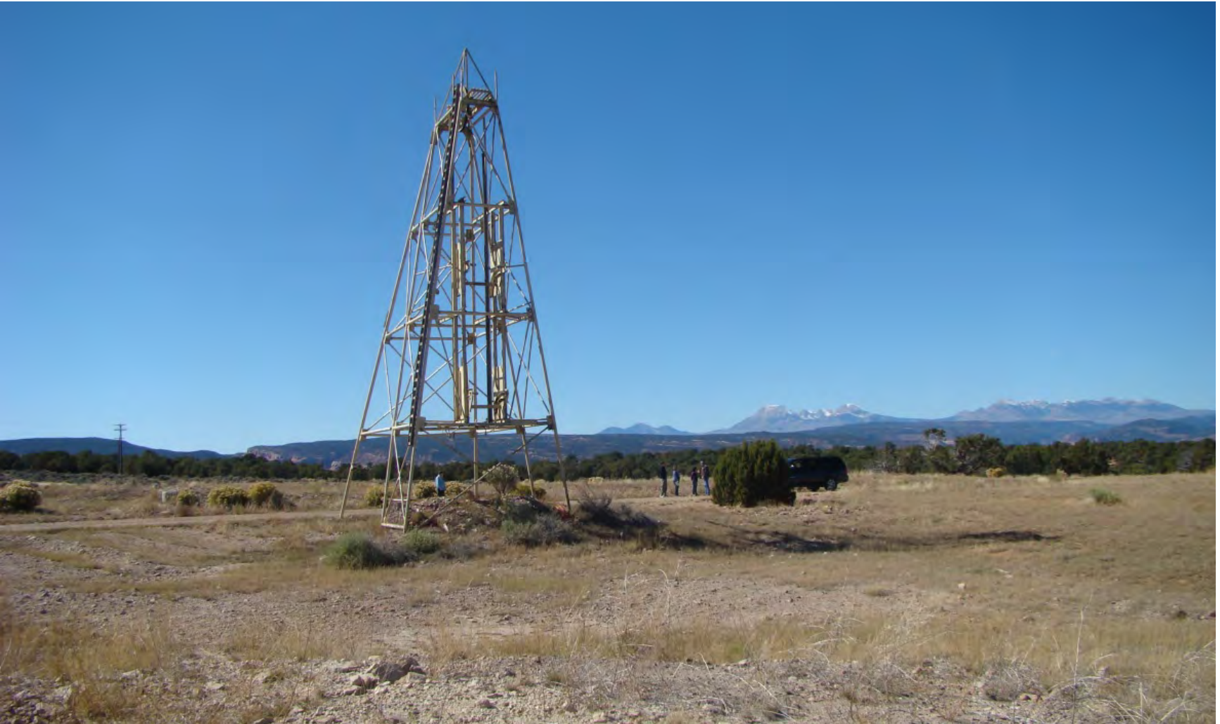
2 FIGURE 3.12-7 View of Lease Tract 19 Facing West (A headframe structure is located above the closed shaft of the Golden Cycle 3 underground mine.)
