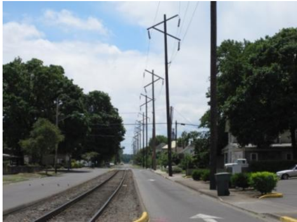
View 11: View from Territorial Street and 4th Street, looking south
