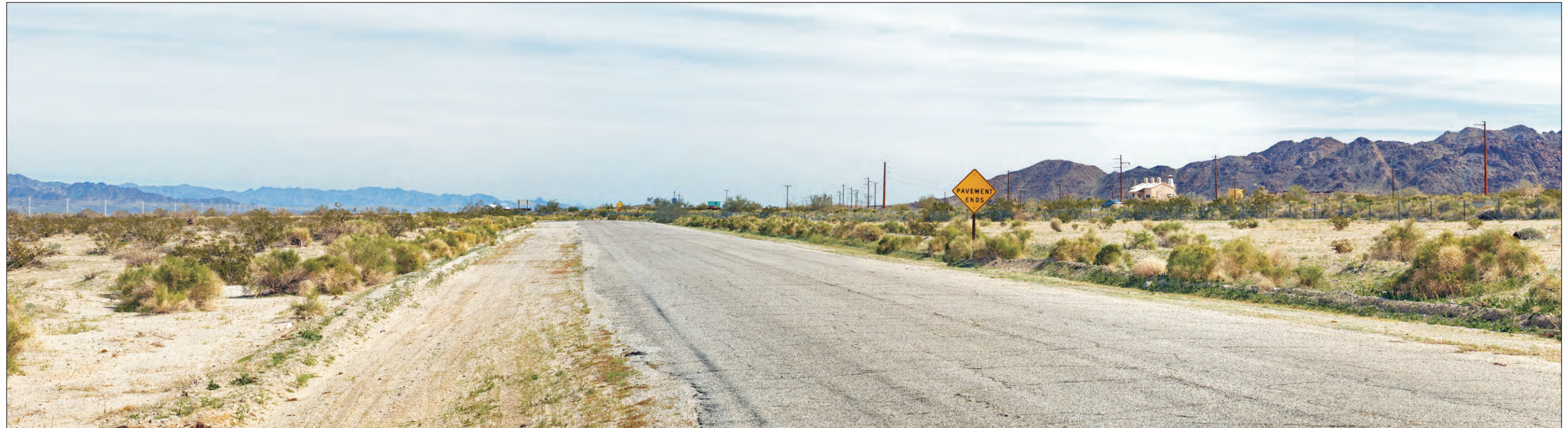
Visual simulation depicting Gen-Tie line A-1 approximately 0.75 of a mile north of Ragsdale Road with Interstate 10 crossover to Red Bluff Substation.
