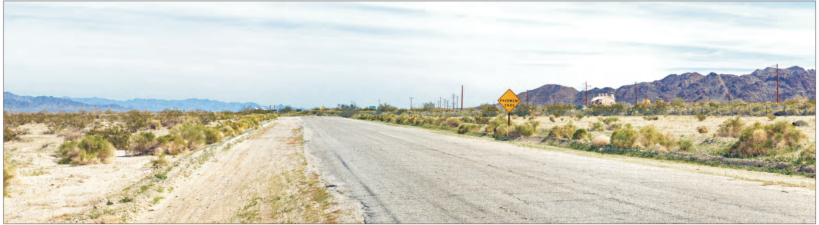
View east along Ragsdale Road showing existing conditions, Desert Center, California.
