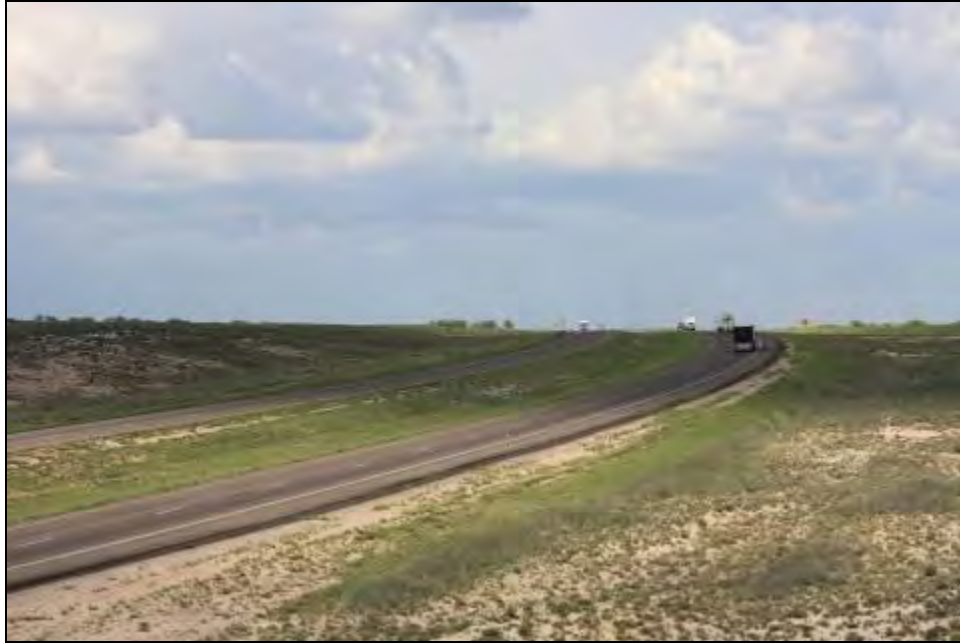
Figure 3.19. Eastbound viewshed along Interstate 20 at the junction with Farm-to-Market Road 1053.
