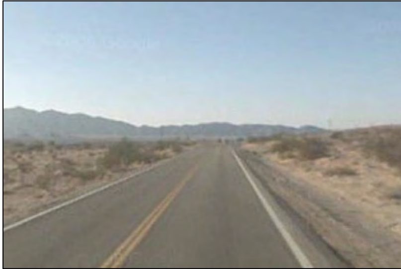
Figure 3-5 View of SR 72 east of the junction with SR 95.
