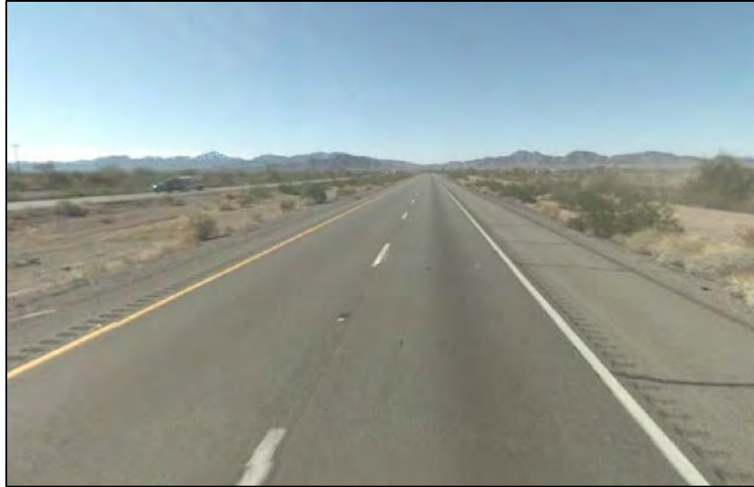
Figure 3-3 View of I-10 east of Quartzsite facing west.
