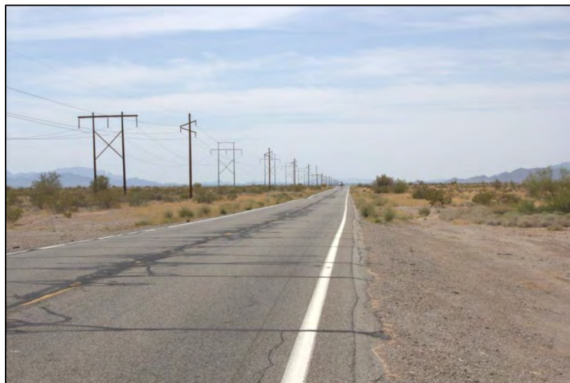
Figure 3-4 View of SR 95 adjacent to the Project area facing south.
