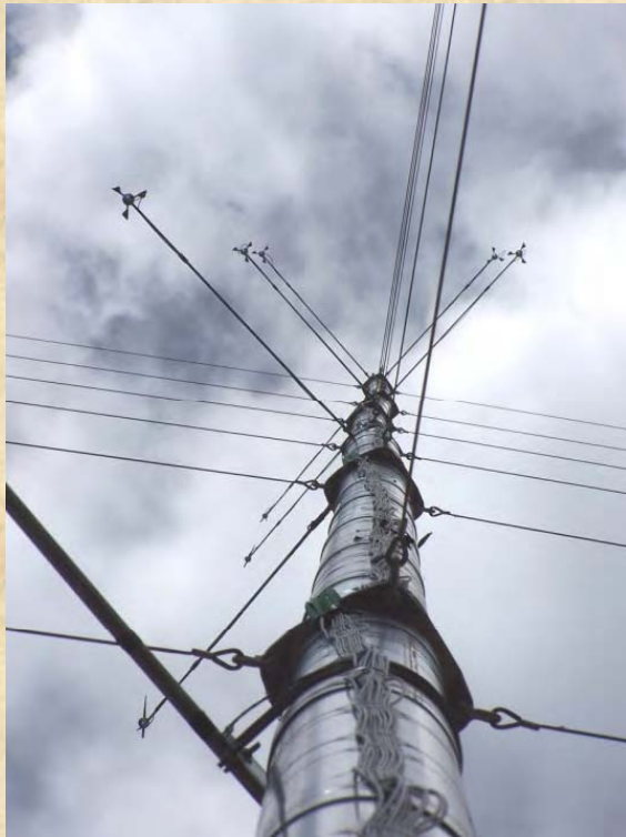
Typical Meteorological “MET” Tower
