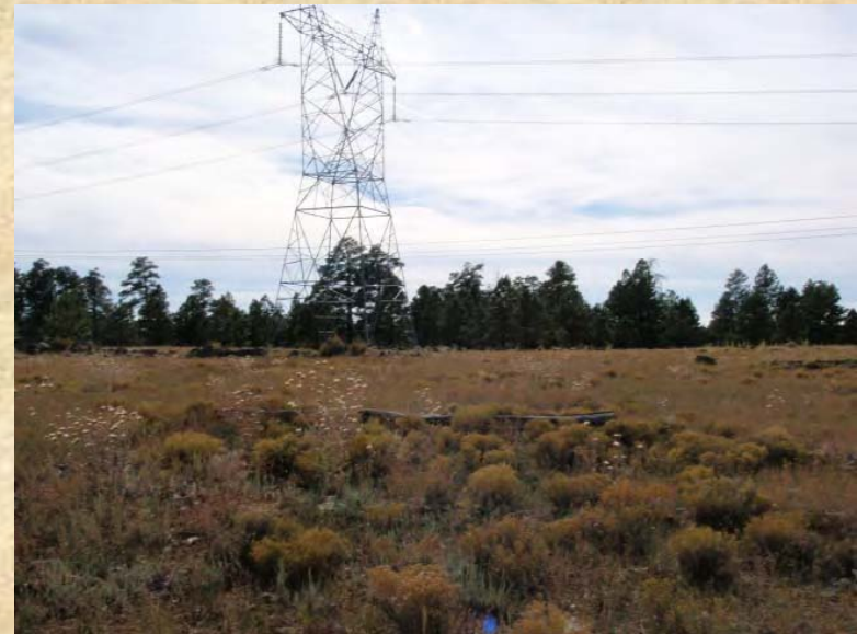
Above: Existing Western Transmission Line, Potential Interconnection Area. Left, an existing 345kV switchyard
