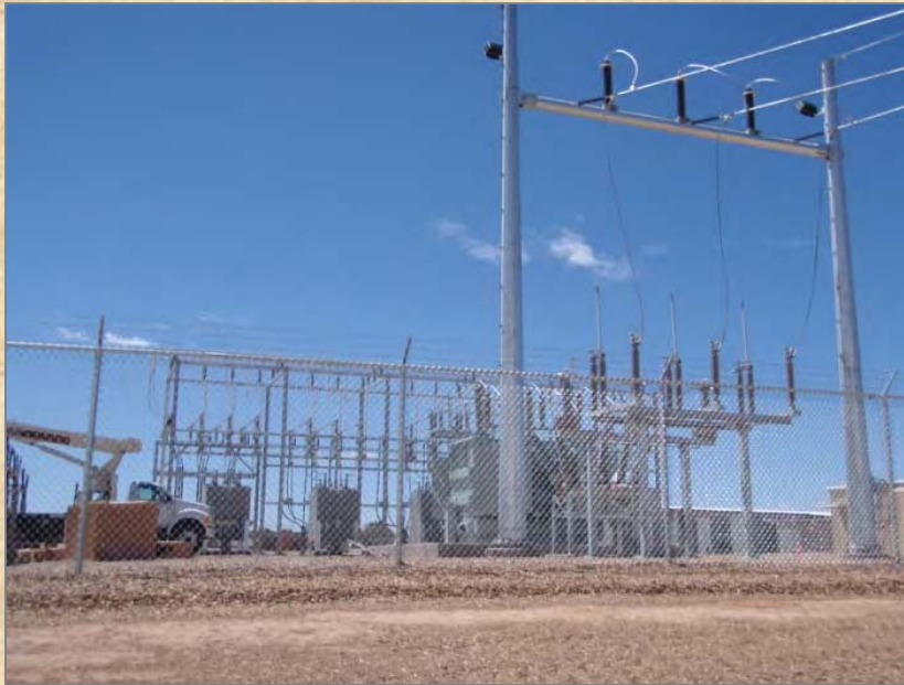
Above: Typical Step-up Substation
