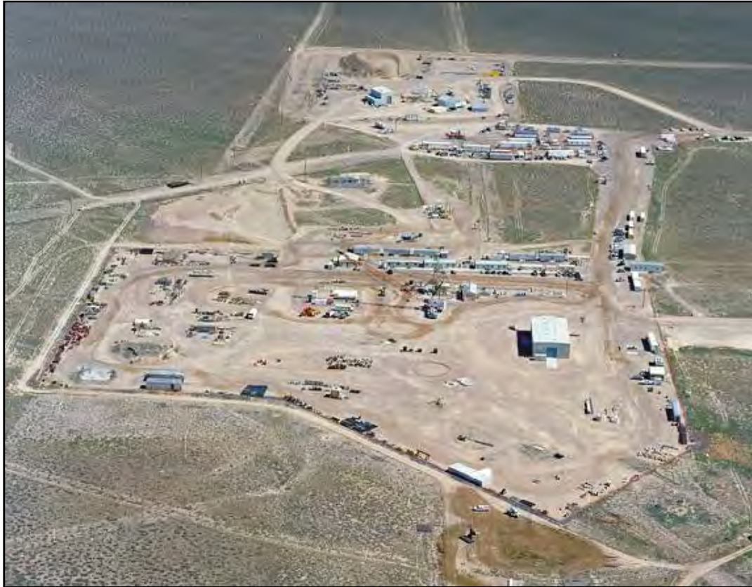
Figure 2-3 Aboveground Facilities of the U1a Complex
