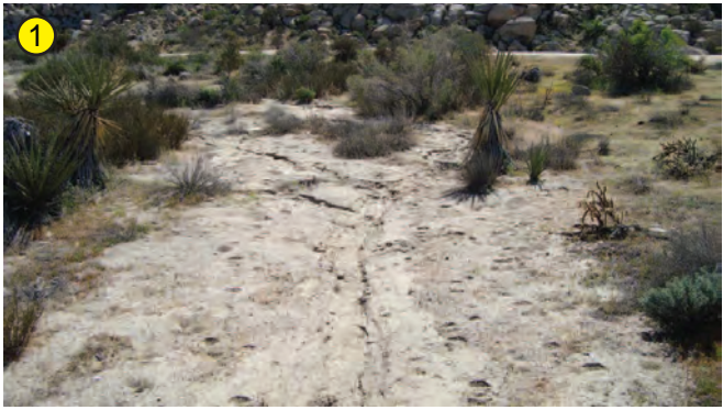
View of southern erosive feature looking east, with roadway in top background.
