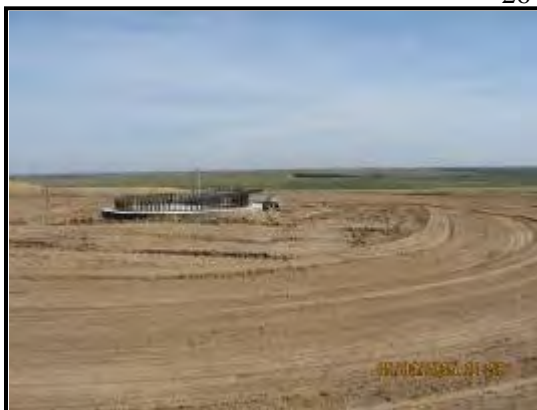
Figure 2.3-8. Typical WTG Spread Foundation During Construction
