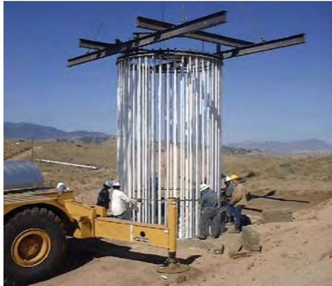
1 2 3 4 5 6 7 8 9 10 11 12 13 14 15 16 17 18 19 20 21 22 23 24 25 26 27 FIGURE 3.3-2 Installation of Turbine Pier Foundation (Source: Photo courtesy of RES Americas. See http://www.res-americas.com for more details.)
