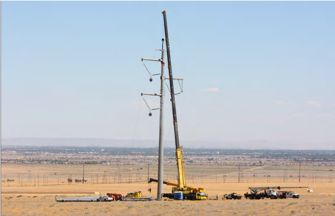
2 FIGURE 5.7-2 Transmission Structure under Construction
