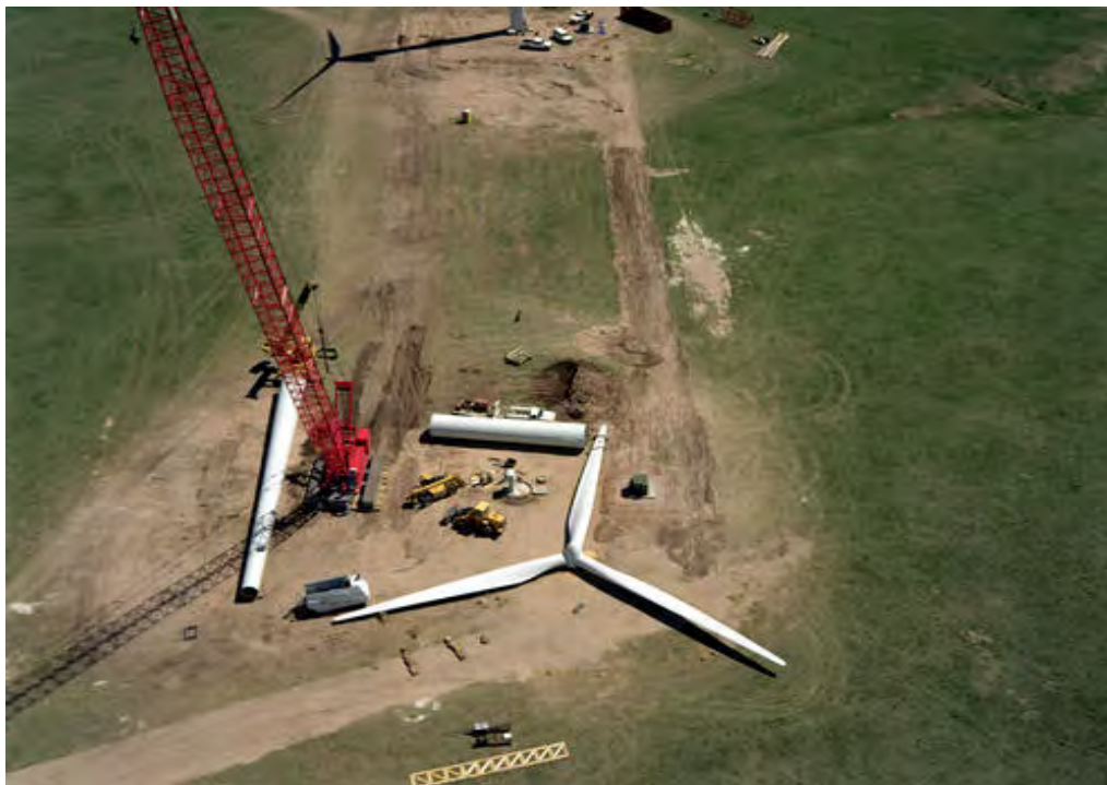
1 2 FIGURE 3.3-3 Aerial View of Preparations to Erect a Wind Turbine Tower at the 3 Public Service of Colorado Ponnequin Wind Farm, Weld County, Colorado 4 (Source: NREL 1999. Photo credit: Warren Getz) 5 6
