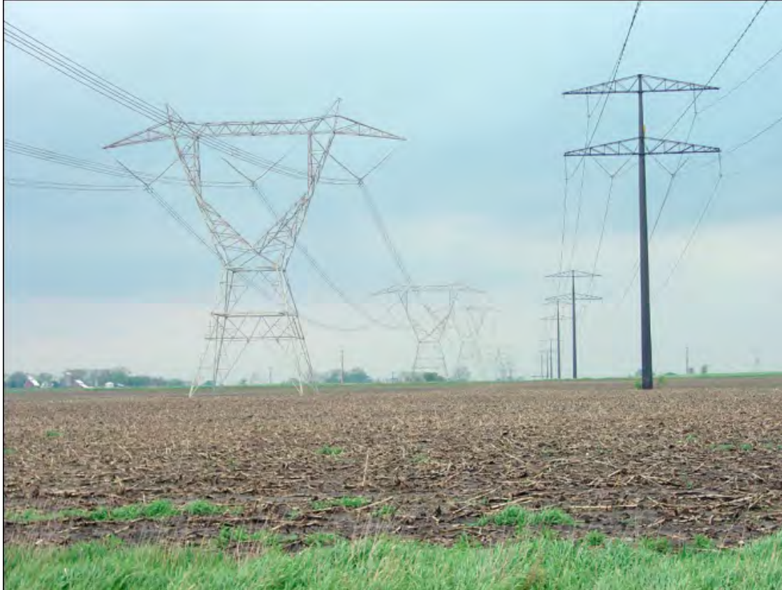
FIGURE 5.7-3 Transmission Structures: Lattice (left) and Monopole (right)
