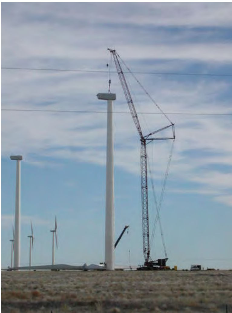
1 2 FIGURE 3.3-4 Wind Turbine Nacelle Installation at Golden 3 Prairie Wind Farm, Lamar, Colorado (Source: NREL 2003. 4 Photo credit: David Jager) 5 6
