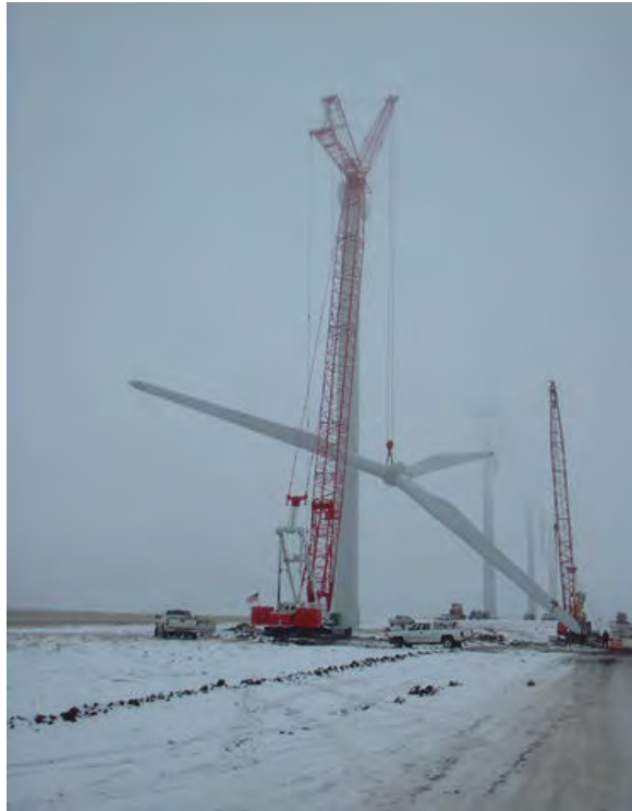
FIGURE 3.3-5 Installation of a Rotor on a General Electric 1.5-MW Wind Turbine at the Klondike, Oregon, Wind Farm (Source: NREL 2002. Photo credit: Paul Woodin)
