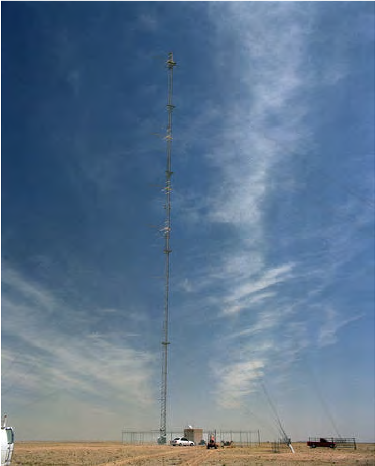
2 FIGURE 5.7-1 394-ft Lattice-Type Guyed Meteorological Tower
