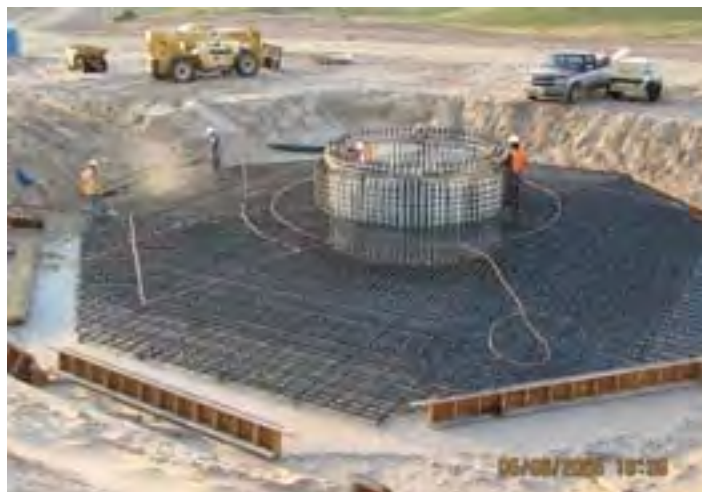
27 28 FIGURE 3.3-1 Turbine Mat Foundation under 29 Construction (Source: Photo courtesy of RES 30 Americas. See http://www.res-americas.com for more 31 details.)
