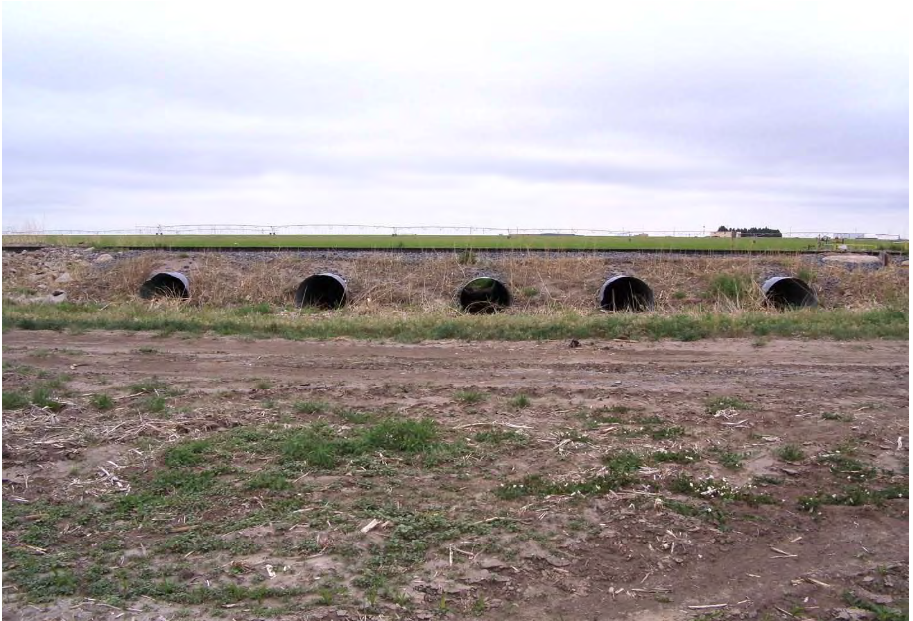
24. Looking south at culverts under railroad tracks along south-central border of the NW 1/4 of Section 17
