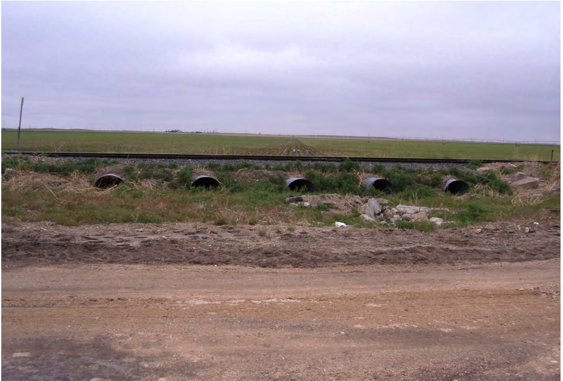
25. Looking north at culverts under railroad tracks along south-central border of the NW 1/4 of Section 17
