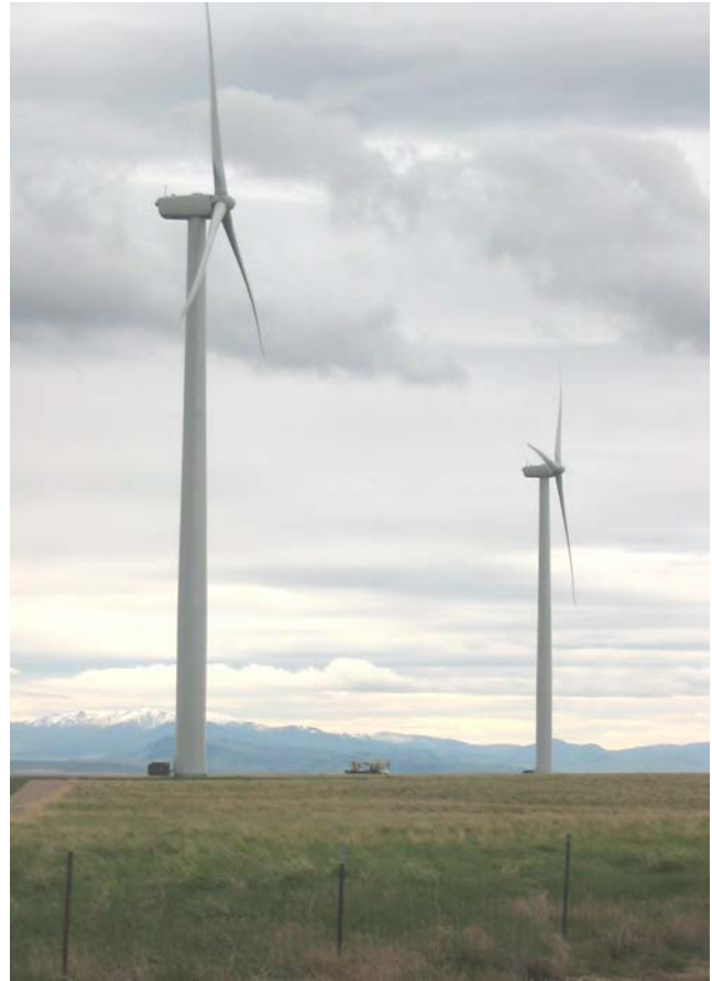
Figure 4.16-1. Two 1.5 MW turbines with passing crane truck and Crazy Mountains in the background.
