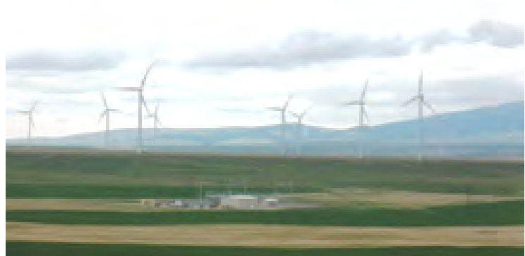
Figure 4.16-3. Judith Gap operations and control facility with foothills of Big Snowy Mountains in the background.
