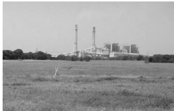
Proposed Jewett Power Plant Site (NRG Limestone Generating Station in the background)
