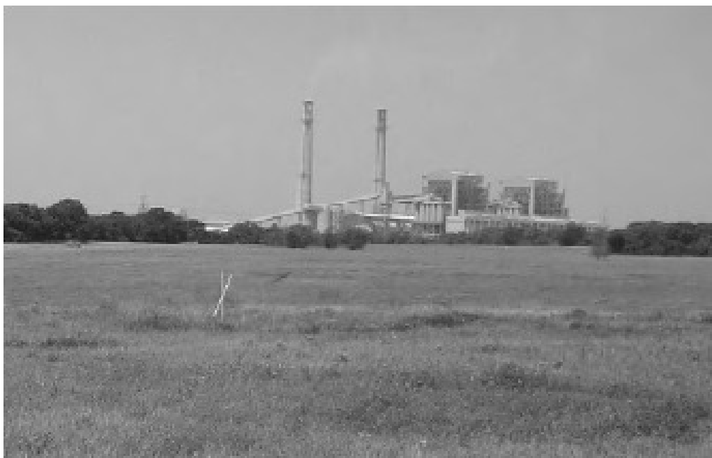
Figure 6.12-1. Proposed Jewett Power Plant Site with NRG Limestone Electric Generating Station in the Background
