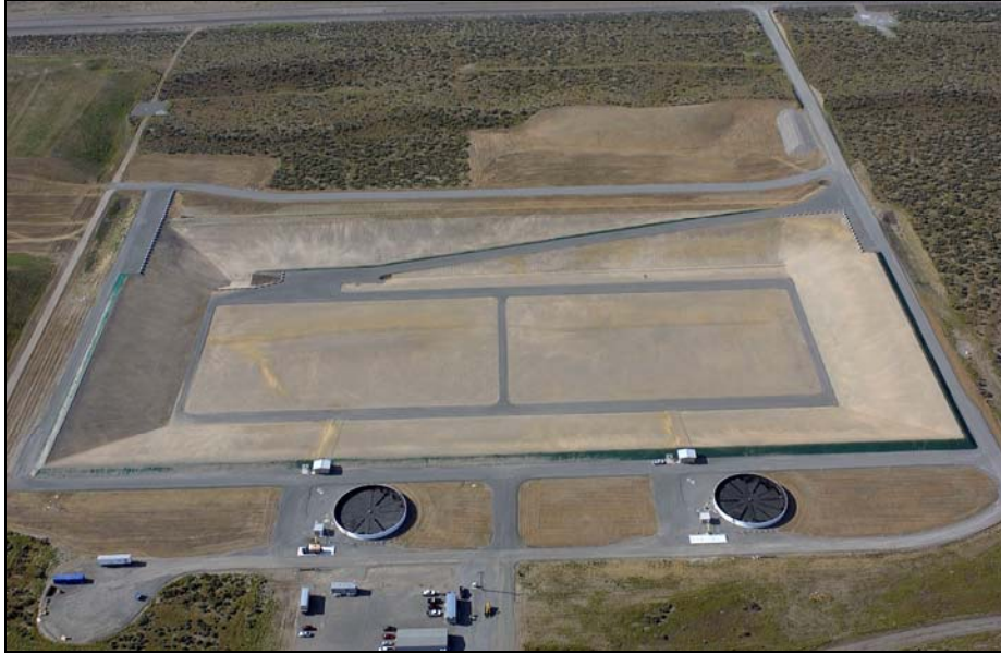
Figure S-11. 200-East Area Integrated Disposal Facility
