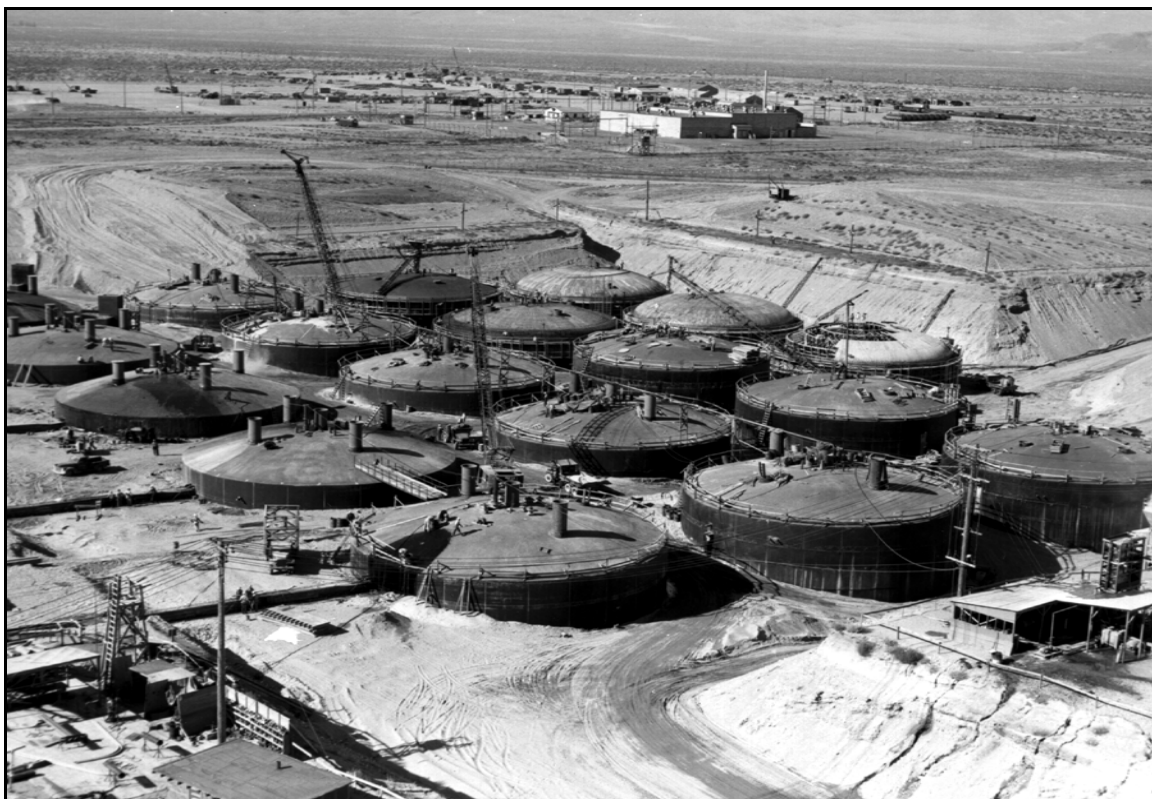
Figure S–2. The Hanford Site’s Waste Tanks Under Construction
