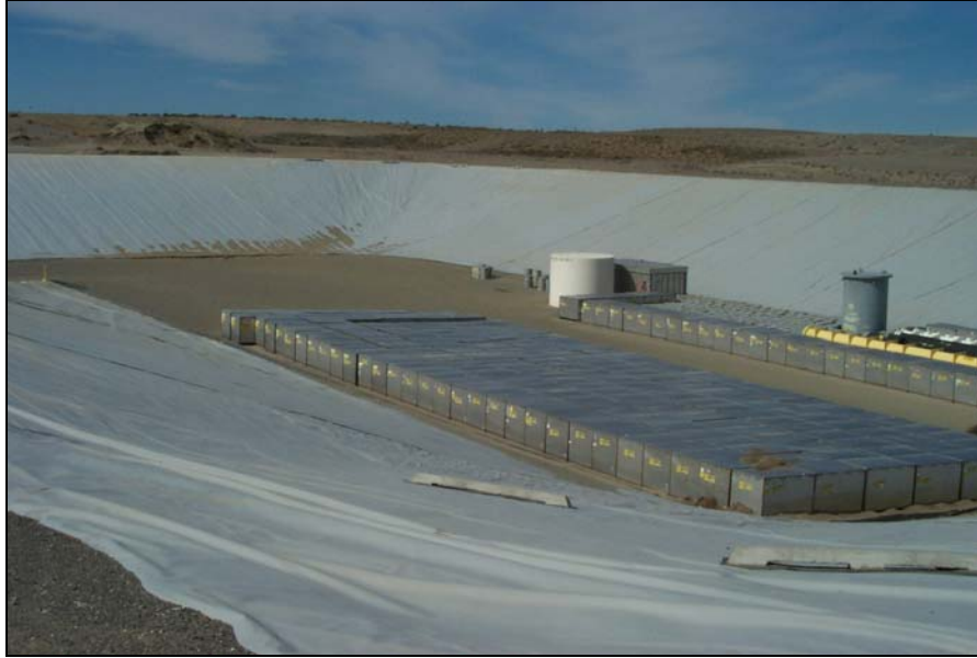
Figure S-7. Low-Level Radioactive Waste Burial Ground Lined Disposal Trench
