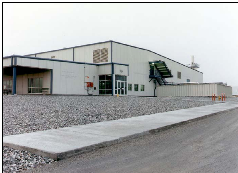
Figure S-10. Waste Receiving and Processing Facility
