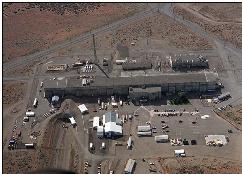
Figure S-9. Aerial View of the T Plant Complex
