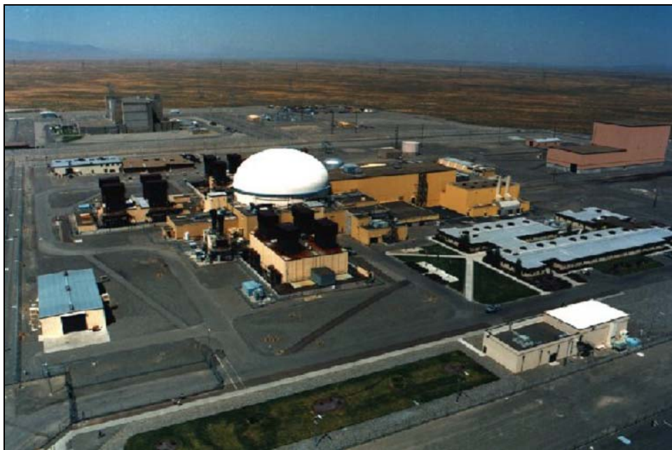
Figure S-6. Fast Flux Test Facility Complex
