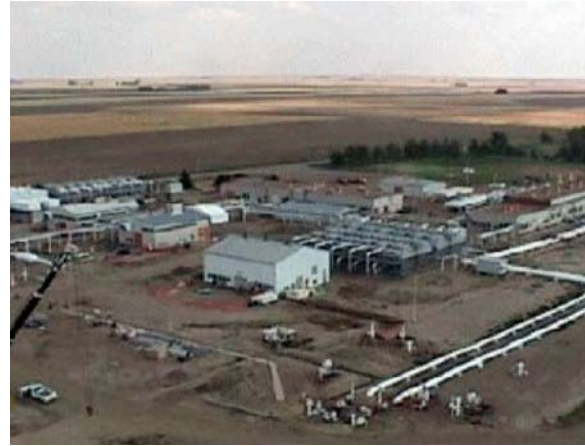
FIGURE 3.9-6 Typical Natural Gas Compressor Station
