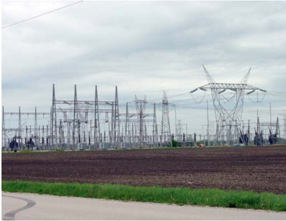
FIGURE 3.9-4 Transmission Lines Leaving Substation
