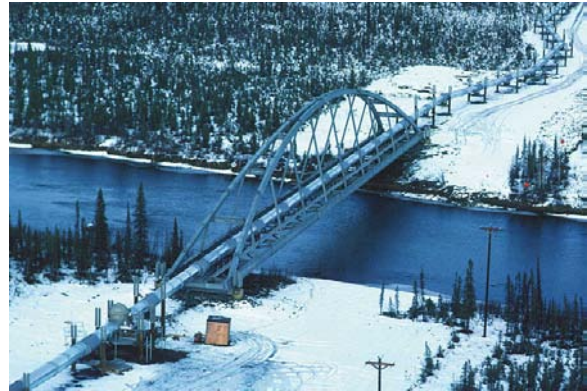
FIGURE 3.9-9 Trans-Alaska Pipeline Bridge over Gulkana River
