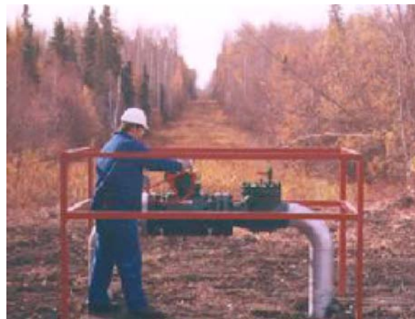
FIGURE 3.9-5 Natural Gas Control Valve
