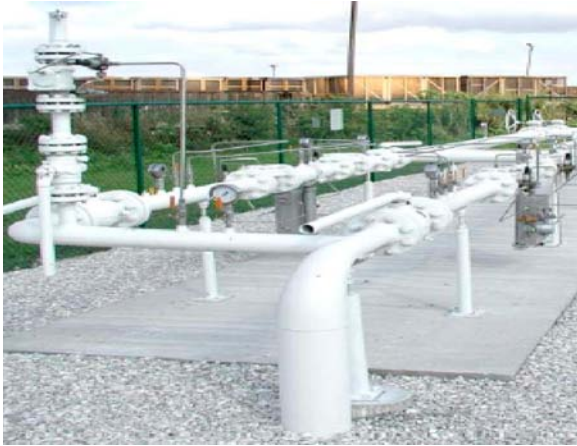
FIGURE 3.9-8 Typical Natural Gas City Gate
