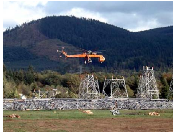
FIGURE 3.9-1 Towers under Construction
